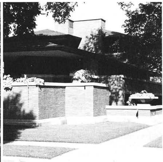
Figure 3.21: Robie House, Chicago
