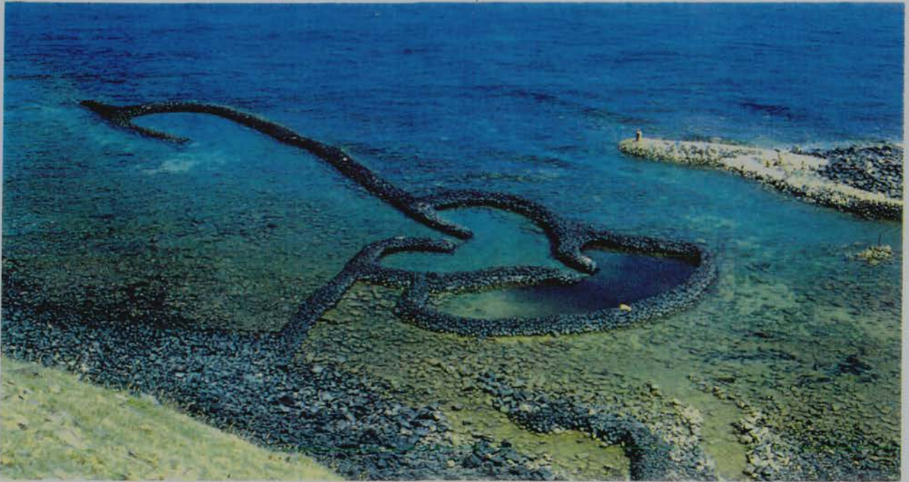
Figure 1-12 General feature of a fish tray (after Tseng, 1987)
