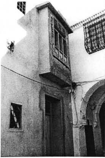
Ill. 2.16a: A modern house in the old city, Tunis, Tunisia; still employing the mashrabiyya , the traditional bay window.
