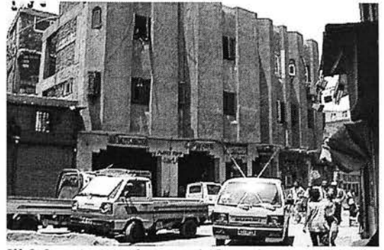
III.2.9: A modern reinforced concrete building, al-Tabbana Street, al-Darb al-Ahmar, see the attempt cope with the historical context using pseudo traditional turned wood fenestration however it came as an ugly interpretation of the heritage due to the lack of architectural guidelines.
