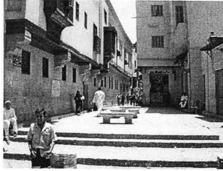
Ill. 6.19: Beautified and restored elevations overlooking al-Darb al-Asfar Street.
