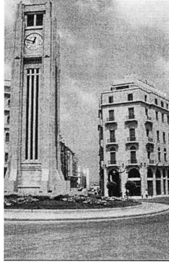
Ill.3.13b: A polished form of Suq Barghout today after being restored and refurbished to accommodate international brand names and very wealthy international community as targeted by the SOLIDERE in charge of the regeneration of the area.
