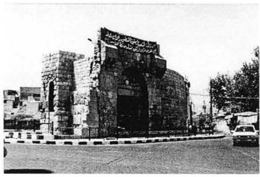
Ill. 1.6b: The old gate in Bab Toma area became a landmark in a major node linking the old fabric of old Damascus with the colonial part surrounding the walls. Damascus, Syria.
