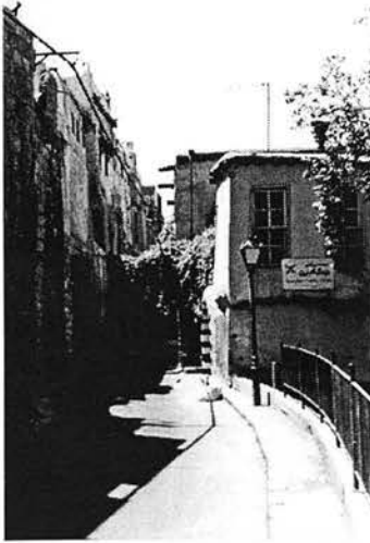
Ill. 1.7a: Houses surmounting walls between Bab Toma gate and Bab al-Salam gate. Damascus, Syria.
