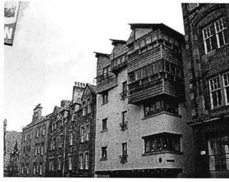
Ill. 3.2: A modern structure in the Royal Mile, the Old Town in Edinburgh; it is not necessary to build an old-looking structure within historical areas to safeguard their integrity, yet it needs much creativity to complement the historical context visually without compromising the contemporary needs.
