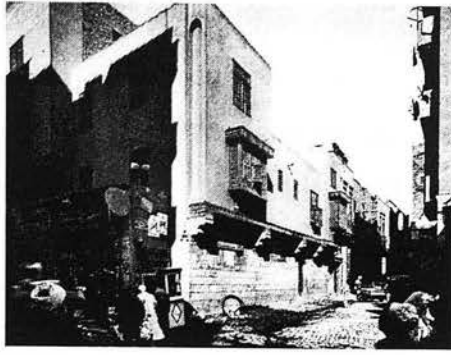
Ill. 6.16a: The old shops along Mustafa Gafar wall on al-Muiz Street; a shot taken in 1970s.
