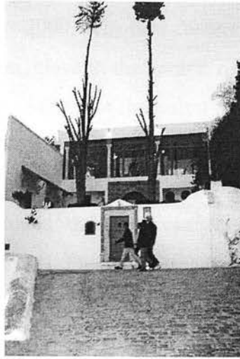
Ill. 3.12a: A historic house converted into a restaurant in Sidi Bu Said, Tunis, Tunisia.
