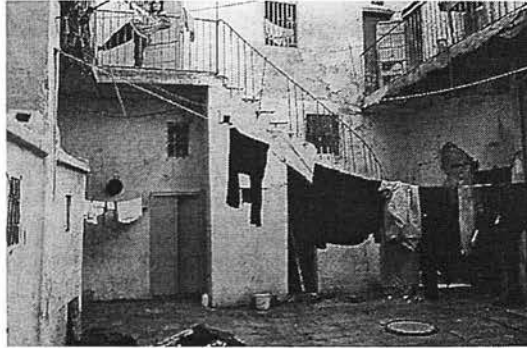
Ill. 3.8a: A court of a historical mansion in le-Median (historic town) in Tunis suffer much deterioration, a typical case of historical mansion that used to be the house of well-to-do Tunisian extended families; now accommodating poor immigrants and settlers from the countryside.
