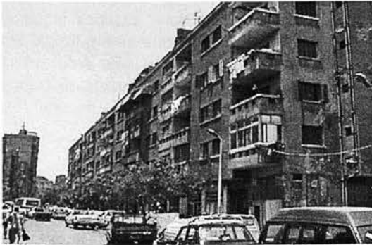
III.2.3: An economical housing scheme built in 1960s, Ahmed Mahir Street, al-Darb al-Ahmar. A drastic dilution of the original character of the historic area emphasised by a development that is launched by the government.
