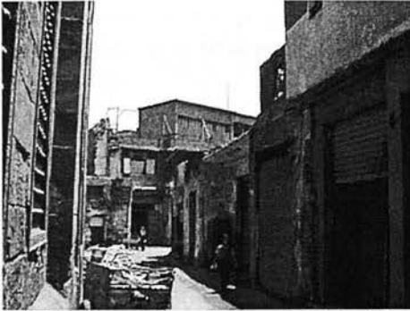
III.2.2: A traditional lane behind Qijmas Mosque, al-Darb al-Ahmar, see the 1960s governmental building contradicting with the context.
