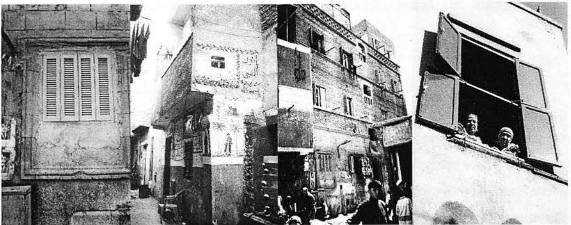
Illustration (A3.2) Cases from al-Darb al-Ahmar, Cairo where improvements undertaken by the users using available materials, designs and know-how violate the historic integrity of the historic buildings.
