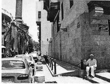
Ill. 6.16b: The western wall of Mustafa Gafar overlooking al-Muiz Street today with all the shops removed and sequenced pavement was paved in a tilted tiling and surrounded with metal chains to prevent any use of it.
