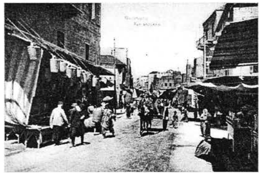
Ill. 1.8b: Suq Barghut area at the turn of the twentieth century, Beirut, Lebanon.
