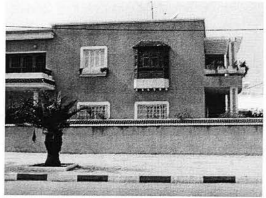
Ill. 2.16b: A modern villa in the suburbs of kairawan, Tunisia; still employing the mashrabiyya , the traditional bay window.
