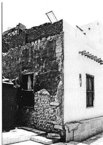
Ill. 6.9a: Superficial urban beautification plastering and painting only the elevation overlooking the main routes in Qasr al-Sham.
