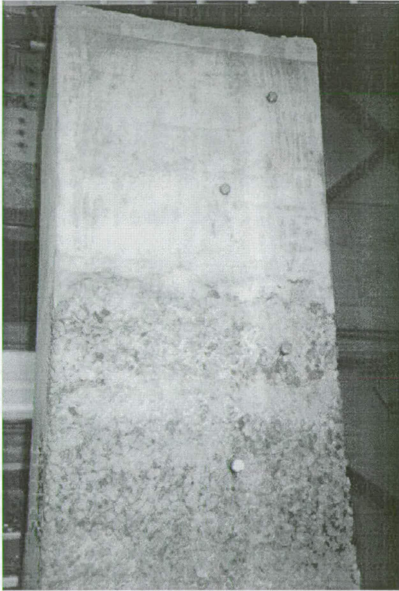
Plate 6.3 Concrete column: transition from 4th to 5th layer
