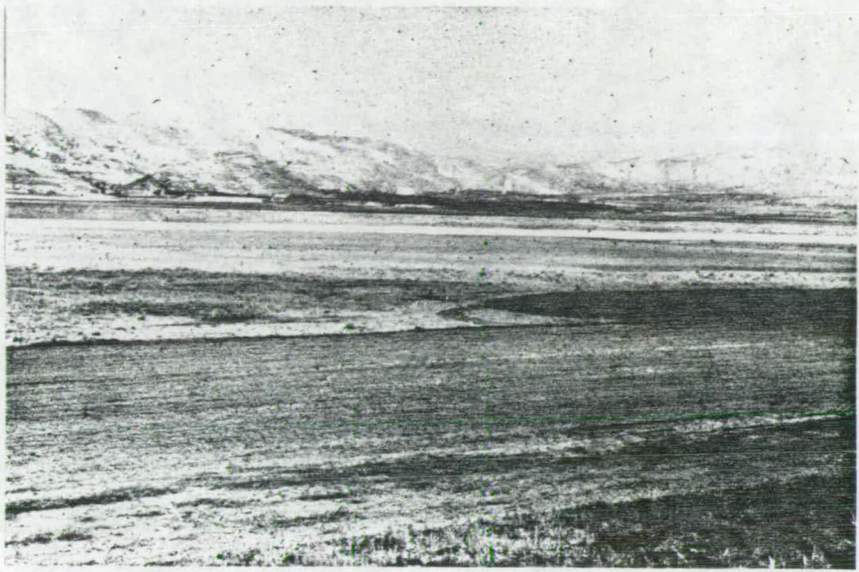
(b) Photo: Shanzhou, near Sanmenxia City, He'nan, 4 August 1980, point A in Figure 3-9. The deposition occupies the whole area in front of the distant hills, with the exception of the reservoir main channel, which may also be seen. (PM)
