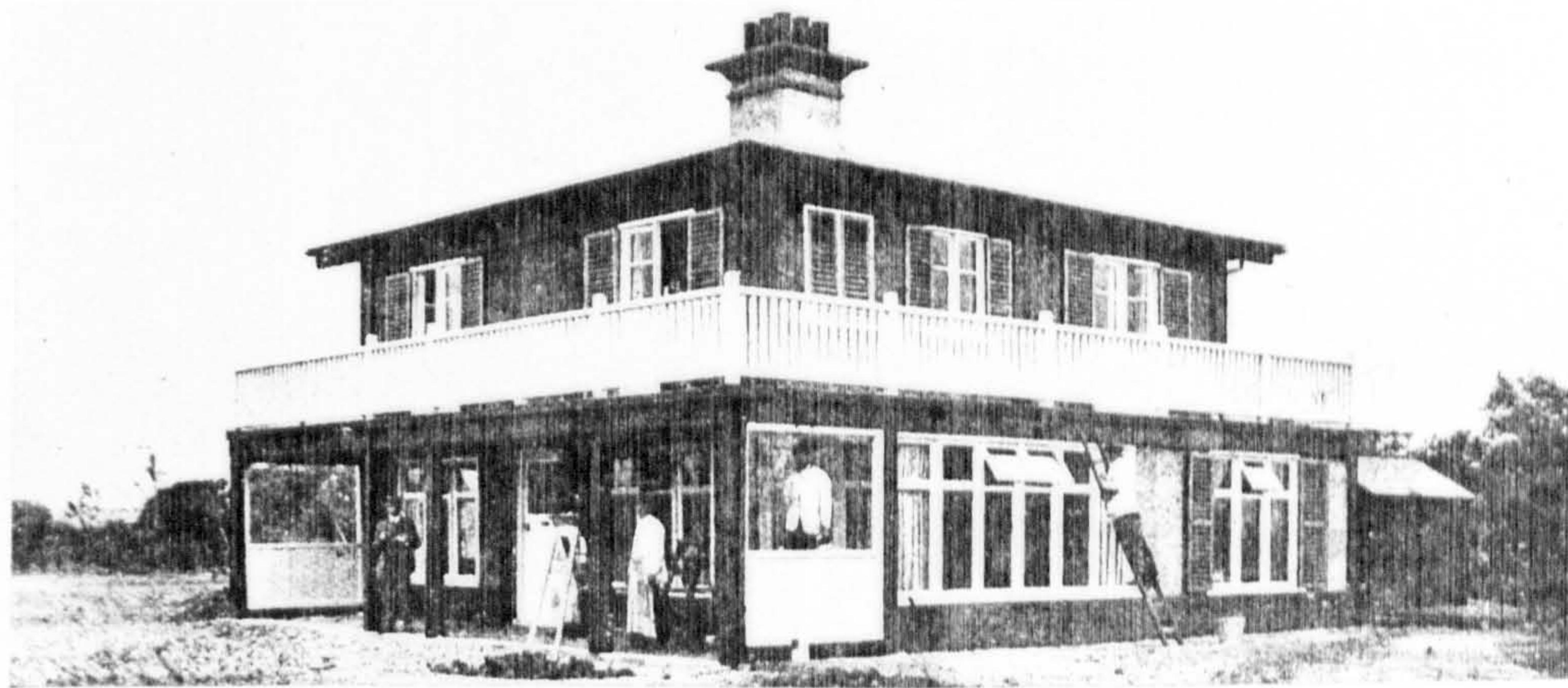
Figure 15: House Fyling Hall: under construction and completed.
