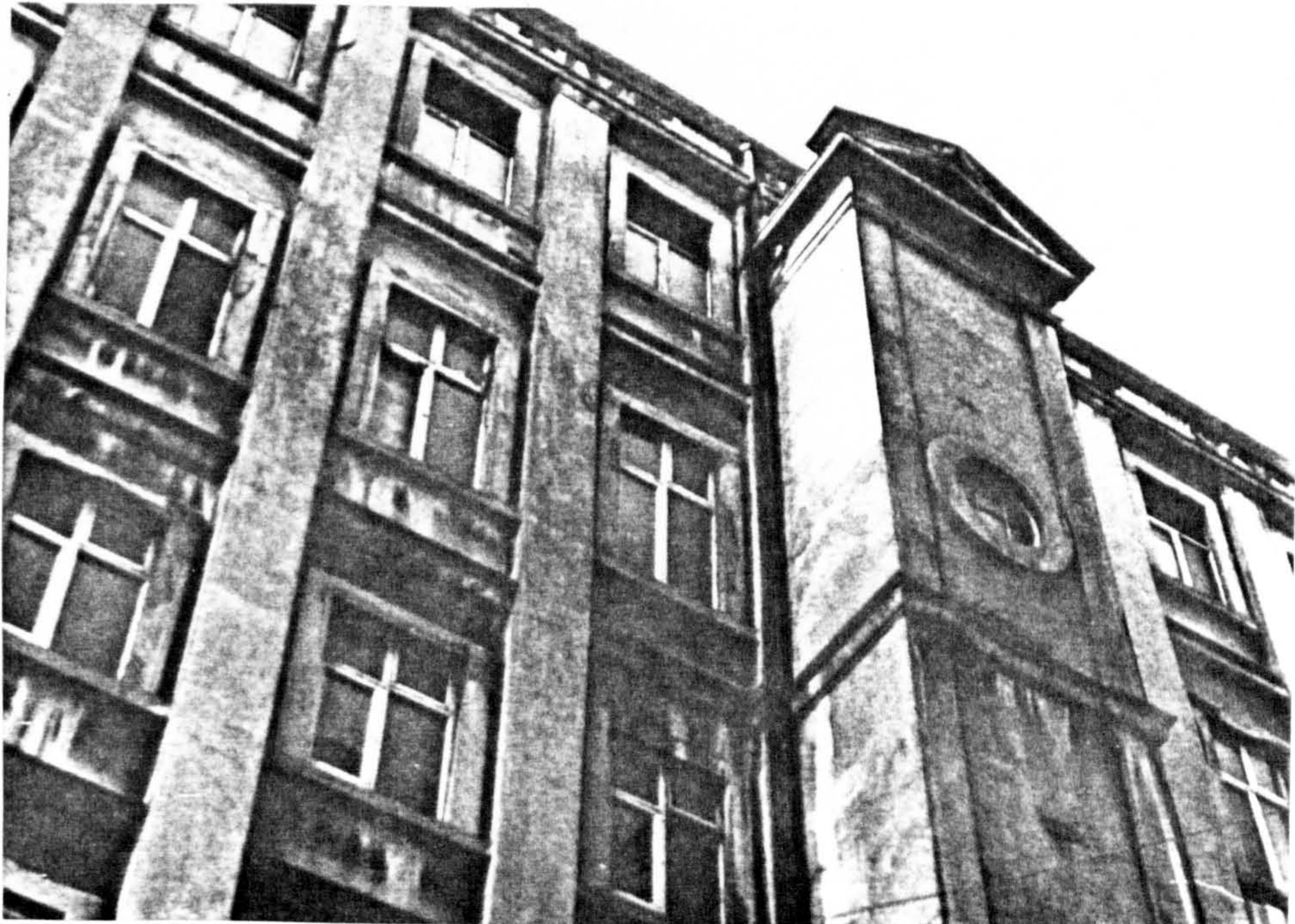
Figure 9: Grain Silos and Cleaning House Dunston: detail.
