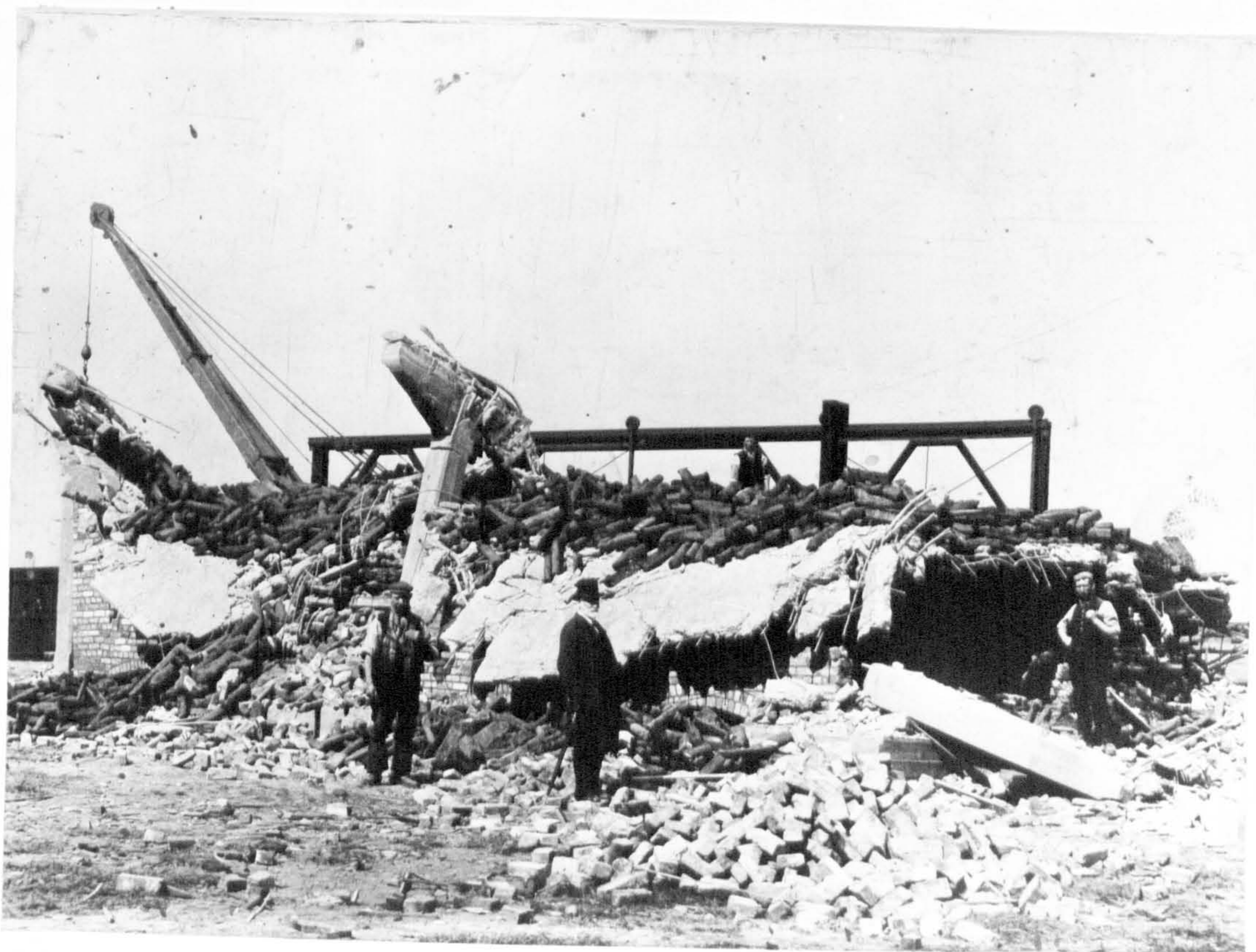
Figure 3: Collapsed test floor.
