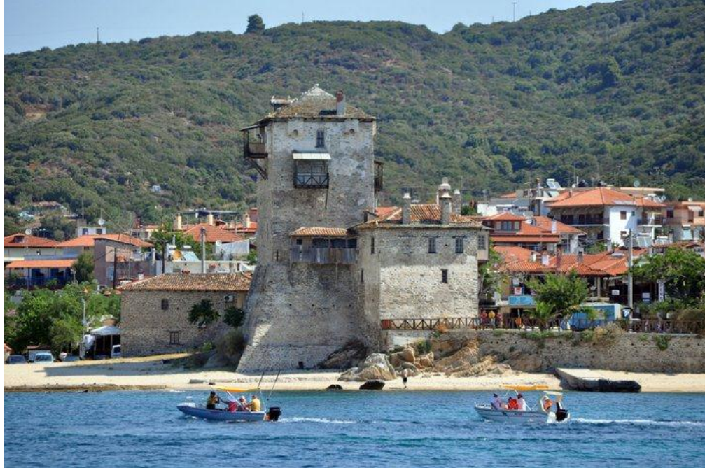
Figure 4.14: The Tower of Ouranoupolis.
