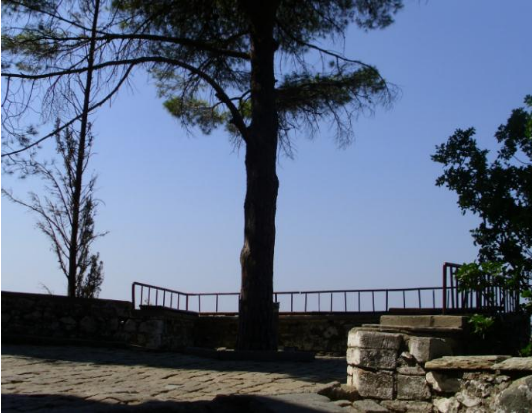
Figures 8.11, 8.12 & 8.13: Ascending the uphill road: the rhythmically planted cypresses and the semi-circular seat.
