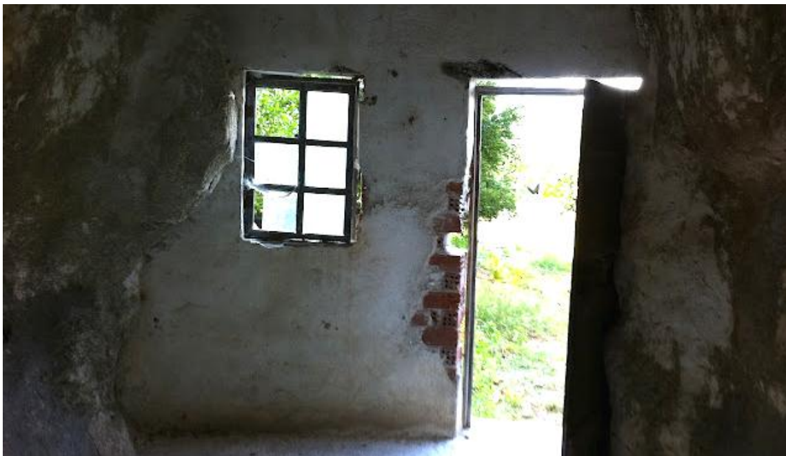
Figure 5.32: The hut in New Skete : The interrelation between the natural cavity and the built boundaries is very intense disclosing this kind of in-between the natural and the artificial.
