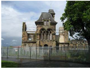
Bellsdyke external view Bellsdyke external view
