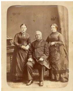
Mr Rhodes Photograph of Mr Rhodes together with his wife and daughter. Believed to have been taken around the time of his inspection of the South Esk Viaduct.
