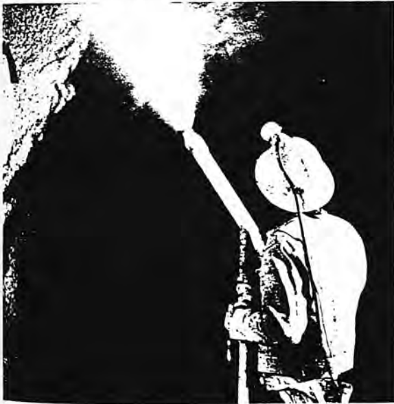
FIG. 1. Shotcreting a tunnel lining.
