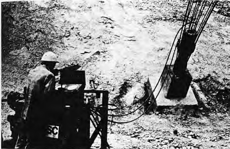
Fig 5. Stressing of Stage 1 Anchor.
