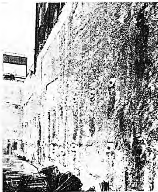
Fig. 9. Close-up view of anchored diaphragm wall—Shepherds Bush
