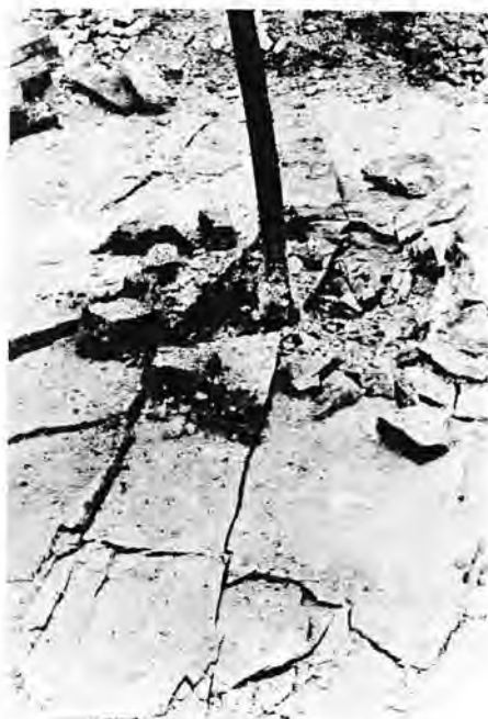
Figure 7 Rock failure strongly controlled by incipient mass structure.
