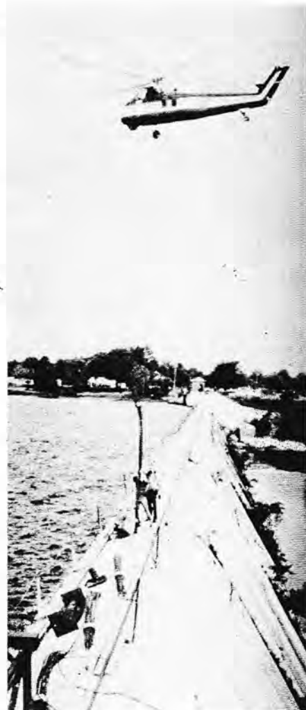
Figure 19 At Milton Dam, Ohio, USA due to difficulty of access, the anchor tendons were transported and homed by helicopter.
