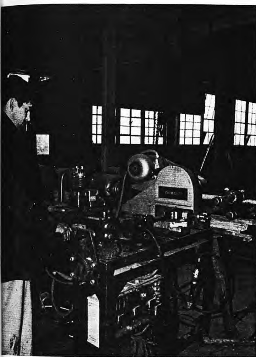
5. Protection of individual strands on site using a specially developed greasing sheathing machine
