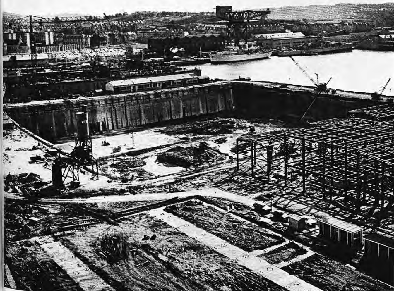
Fig. 1. General view of dewatered basin prior of construction of dry docks at HM Dockyard, Davenport
