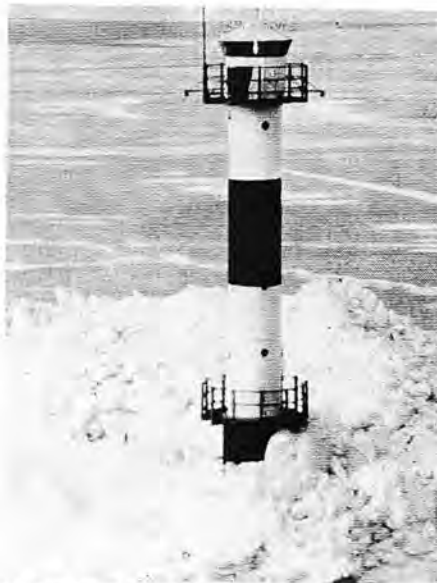
Figure 2 Resistance to sliding and overturning provided by 6 permanent anchors installed in 17m of alluvium and prestressed to 850kN working load, at the lighthouse at Kullagrund on the Baltic coast of Sweden.
