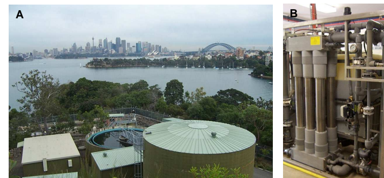
Figure 1 Taronga Zoo water reclamation plant (A) water reclamation plant overlooking Sydney Harbour and (B) microfiltration unit.
