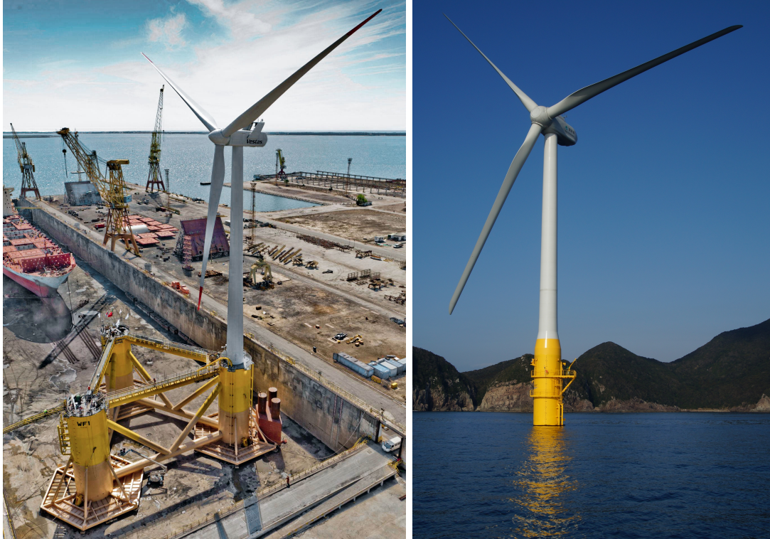
Figure 1.2: WindFloat assembly in the Mitrena Shipyard near Lisbon (left), photo courtesy of Principle Power. Haen-kaze demonstrator sited off Goto in Japan (right), courtesy of David Ingram.
