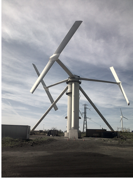
Figure 4.11: Full-scale prototype with 1H rotor, Fos-Sur-Mer, France, 2014. After Dodd [235].
