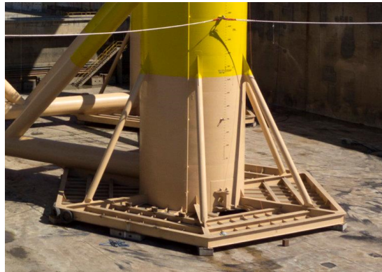
Figure 2.2: Detail of a WindFloat prototype column. Photo courtesy of Principle Power.
