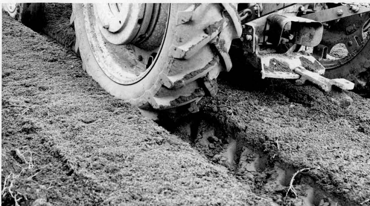
Fig. 11.10 The indication of wheel track compaction on the surface
