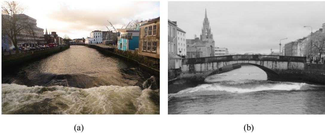
Figure 1.6: Flood wave propagation along the River Lee in Cork, Ireland. Photograph (a) a hydraulic jump as the flow transitions from supercritical to subcritical as it passes a weir, taken from joanfrankham.wordpress.com (b) taken from darkroomdave.com
