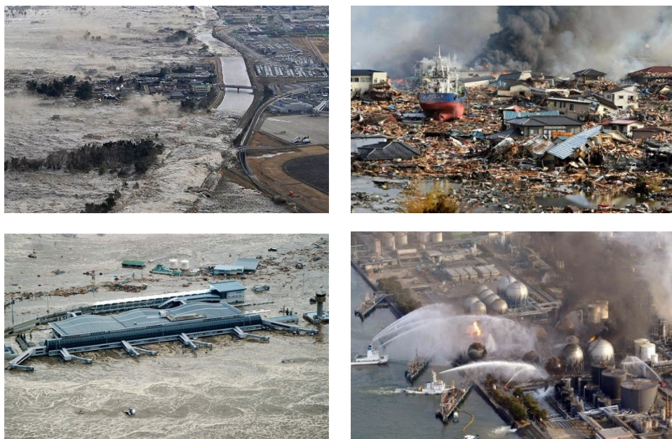
Figure 1.2: Tōhoku tsunami's damages. Photographs of, (a) tsunami wave overtopping sea defences (telegraph.co.uk), (b) destruction at the coastal area (bulicip.comule.com), (c) destruction at the airport (telegraph.co.uk), (d) destruction at the nuclear reactor (prn.fm/tag/fukushima-daiichi-nuclear-disaster/).
