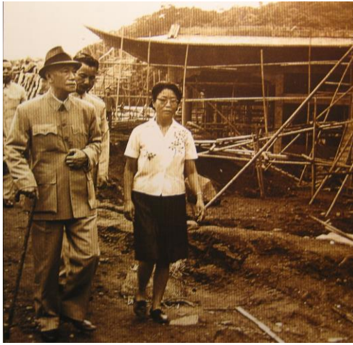
Fig. 6-40 Chiang Kai-shek Oversaw the Construction Site with Architect Siou.
