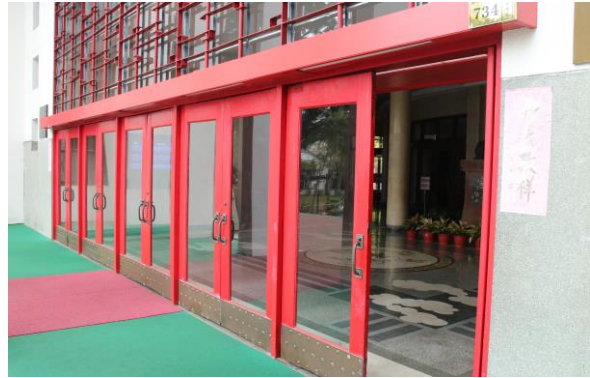
Fig. 6-31 The Main Entrance.
