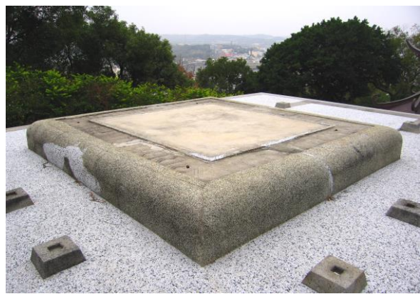
Fig. 4-18 The Demolished Main Hall.
