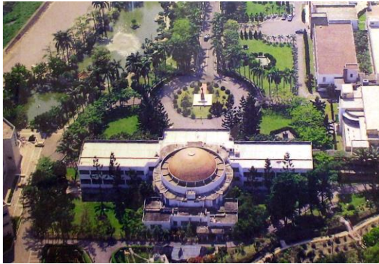
Fig. 6-28 The full View of the Taiwan Provincial Consultative Council Hall.
