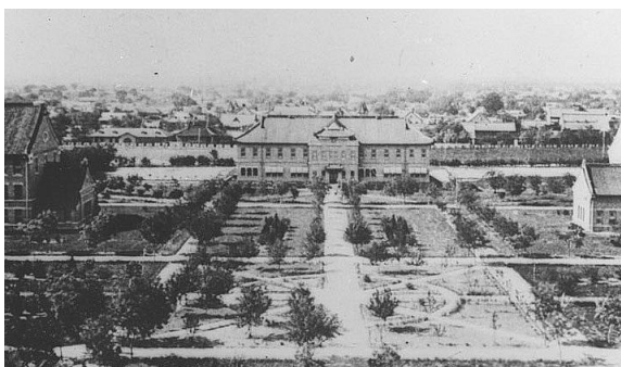
Fig. 3-7 The Administration Building of the Cheeloo University in Shandong.
