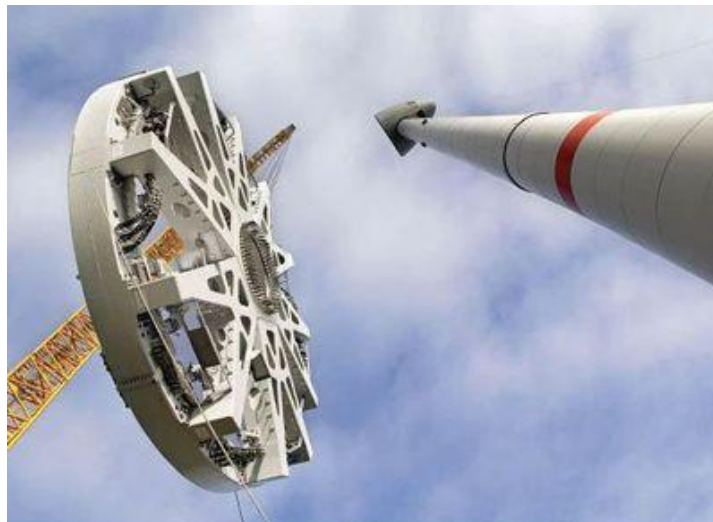
Figure 1.3: Stator assembly of Enercon E126 7.5MW wind turbine (direct drive) generator, (Courtesy of Enercon)
