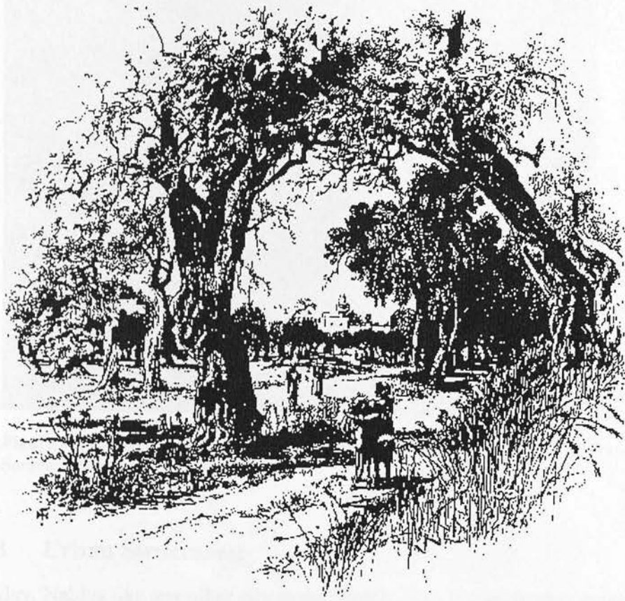
Fig. 4.4 Old photo of Nablus taken from the east entrance.
