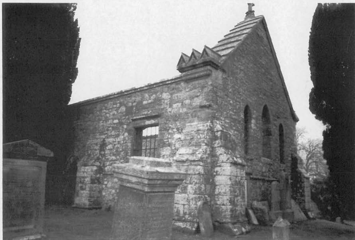
Figure 10.13 Abdie Church, Fife. Original buttresses
