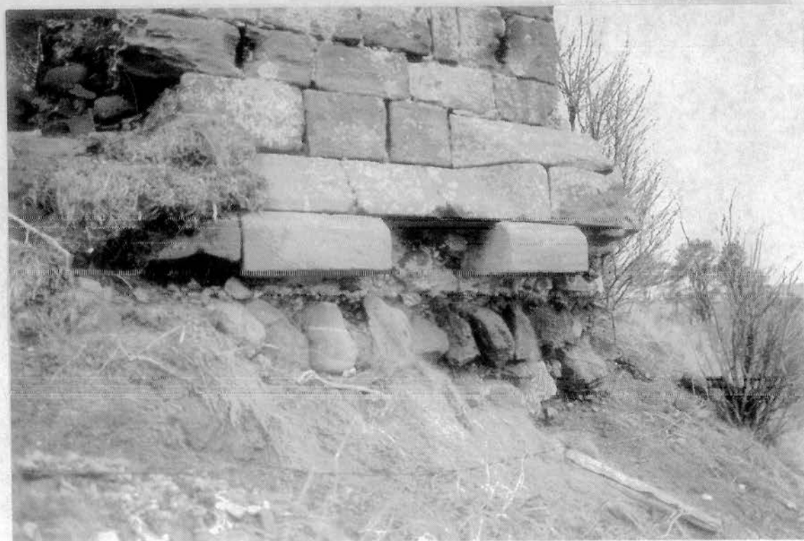
Figure 8.2 Redcastle, Angus. Late 15th century: foundations
