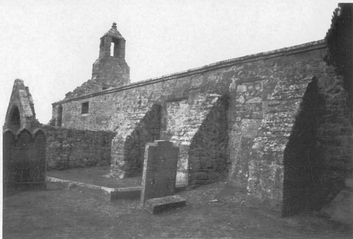
Figure 10.14 Abdie Church. Buttresses added in the 17th century
