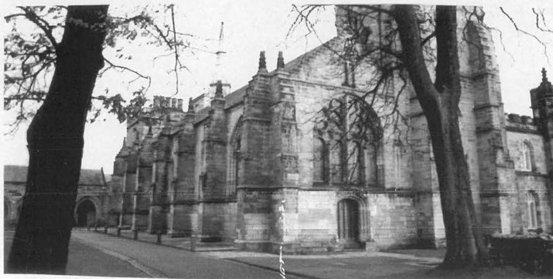
Figure 10.19 King's College Chapel, Aberdeen: top: south cloister elevation bottom: north and west three-quarter view
