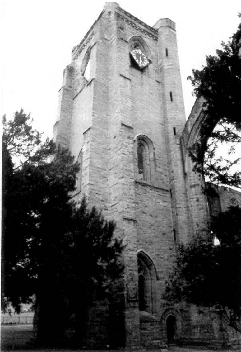
Figure 14.15 Dunkeld Cathedral Tower
