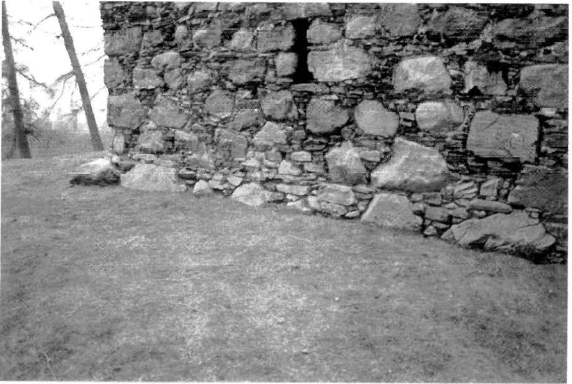
Figure 8.3 Knock Castle, Aberdeenshire. Late 16th century. Boulder foundations
