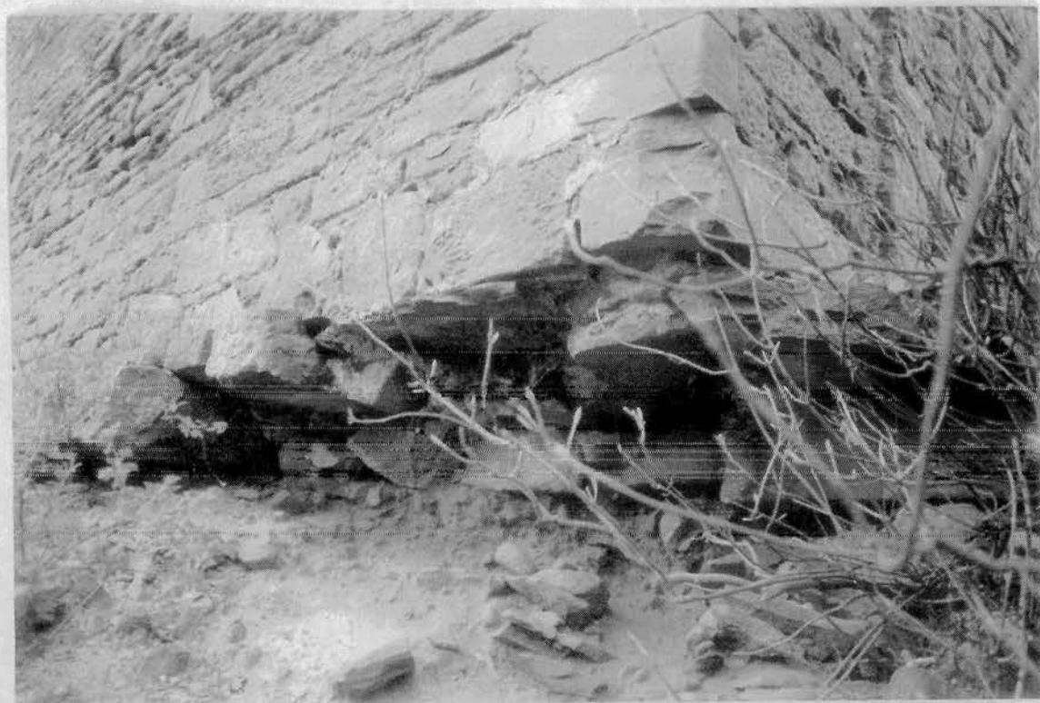
Figure 8.1 Melgund, Angus. Mid 16th century: foundations
