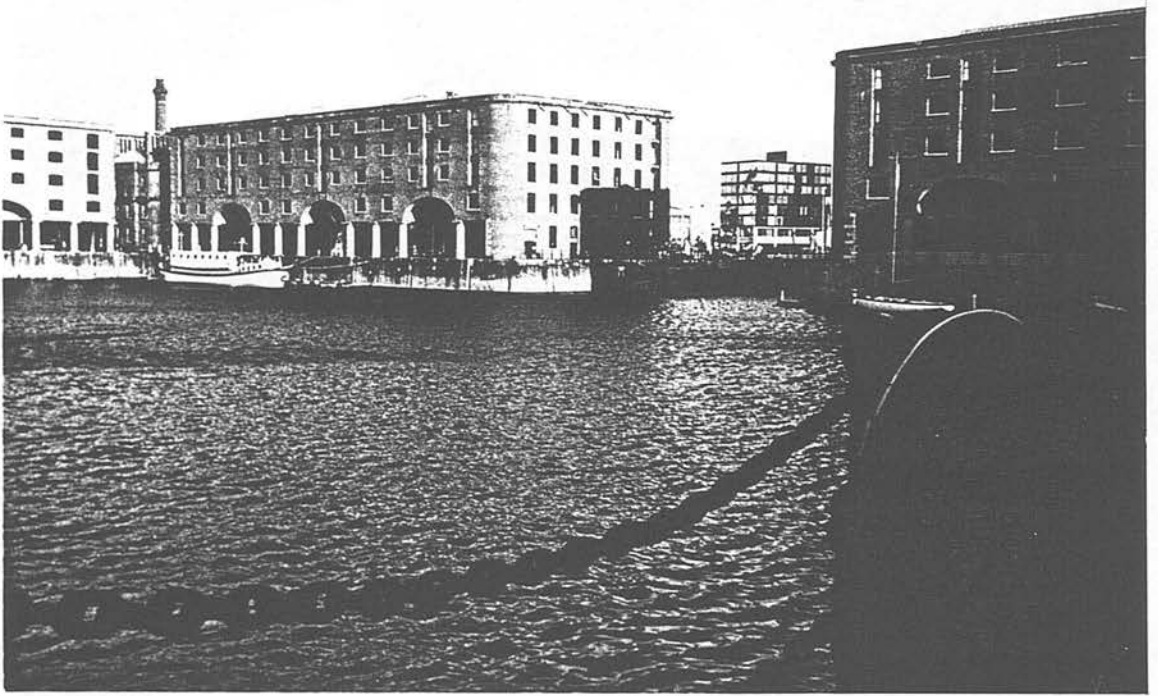
Fig. ( 5.12) Old Albert Dock is converted to cultural commercial centre. It has become the most lively place in Liverpool keeping its cultural continuity.
