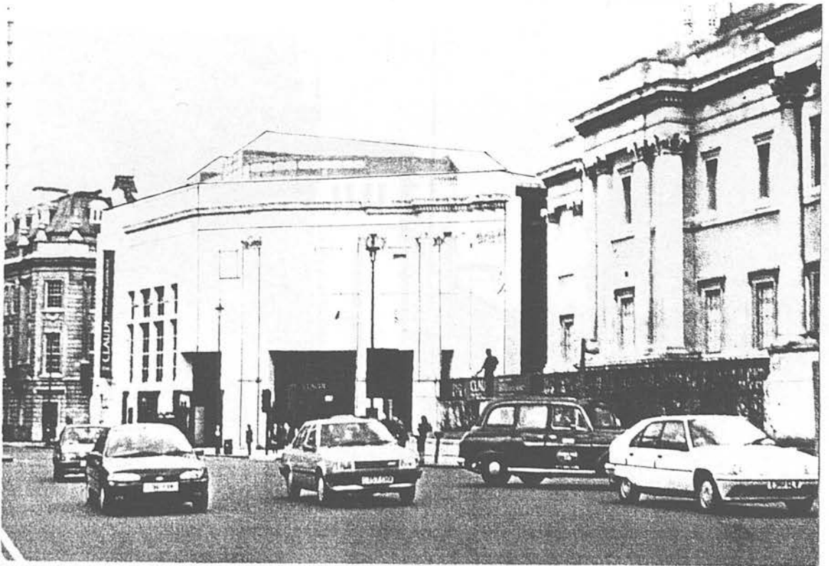
Fig. ( 5.18) The continuity between a historical building and a contemporary one is a main theme of the Sainsbury Wing in relation to the national gallery, London
