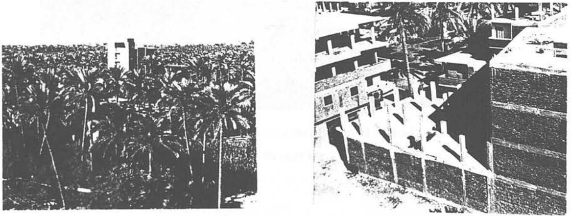
Fig. (1.30) Informal housing sector, Cairo
