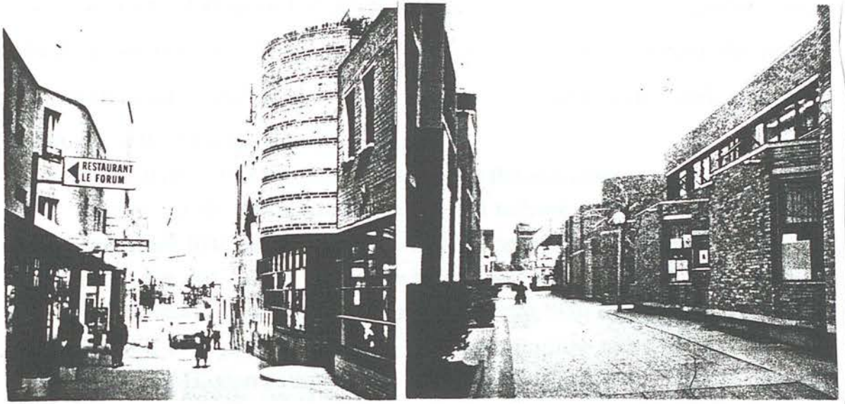
Fig. ( 0.11) Residential scheme, Cergy Pontoise, France
