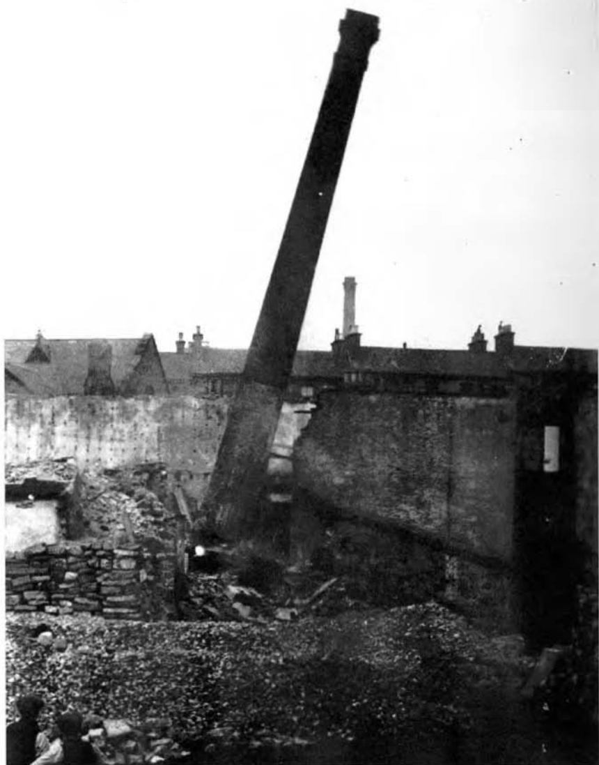
Fig. 5. The Old Summerhall Brewery Chimney being Demolished 23 October 1913 (Royal Dick Archive)
