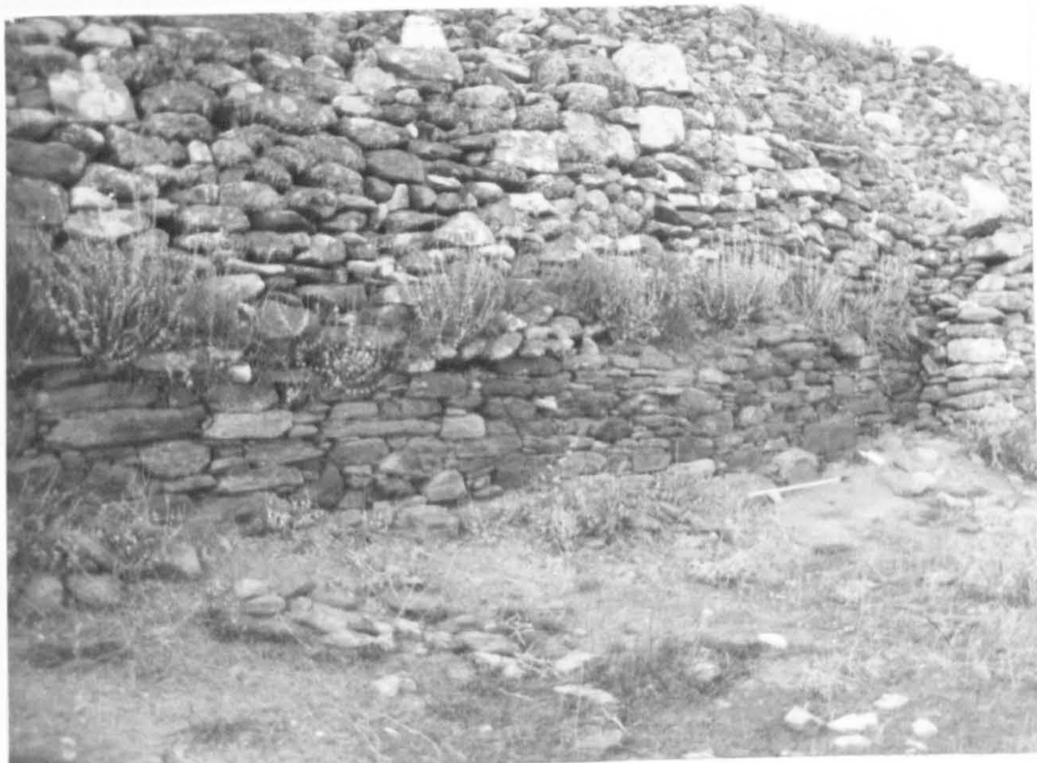
Pl. 65: retaining wall- S part of E wall
