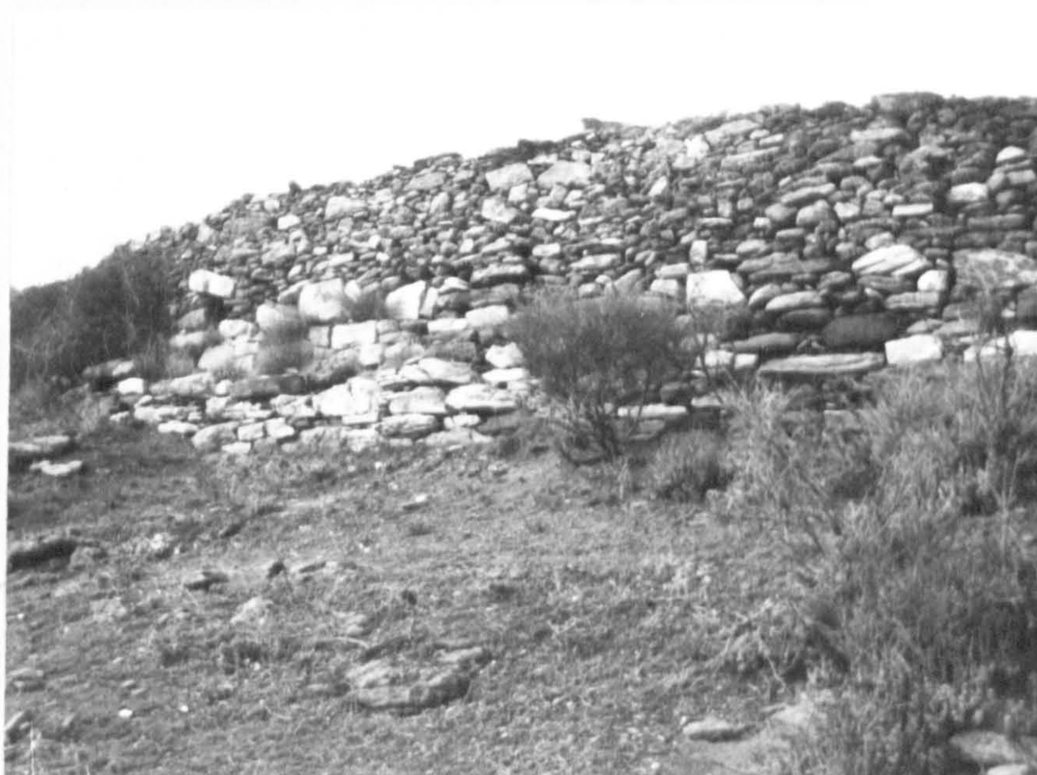
Pl. 66: retaining wall - N part of E wall
