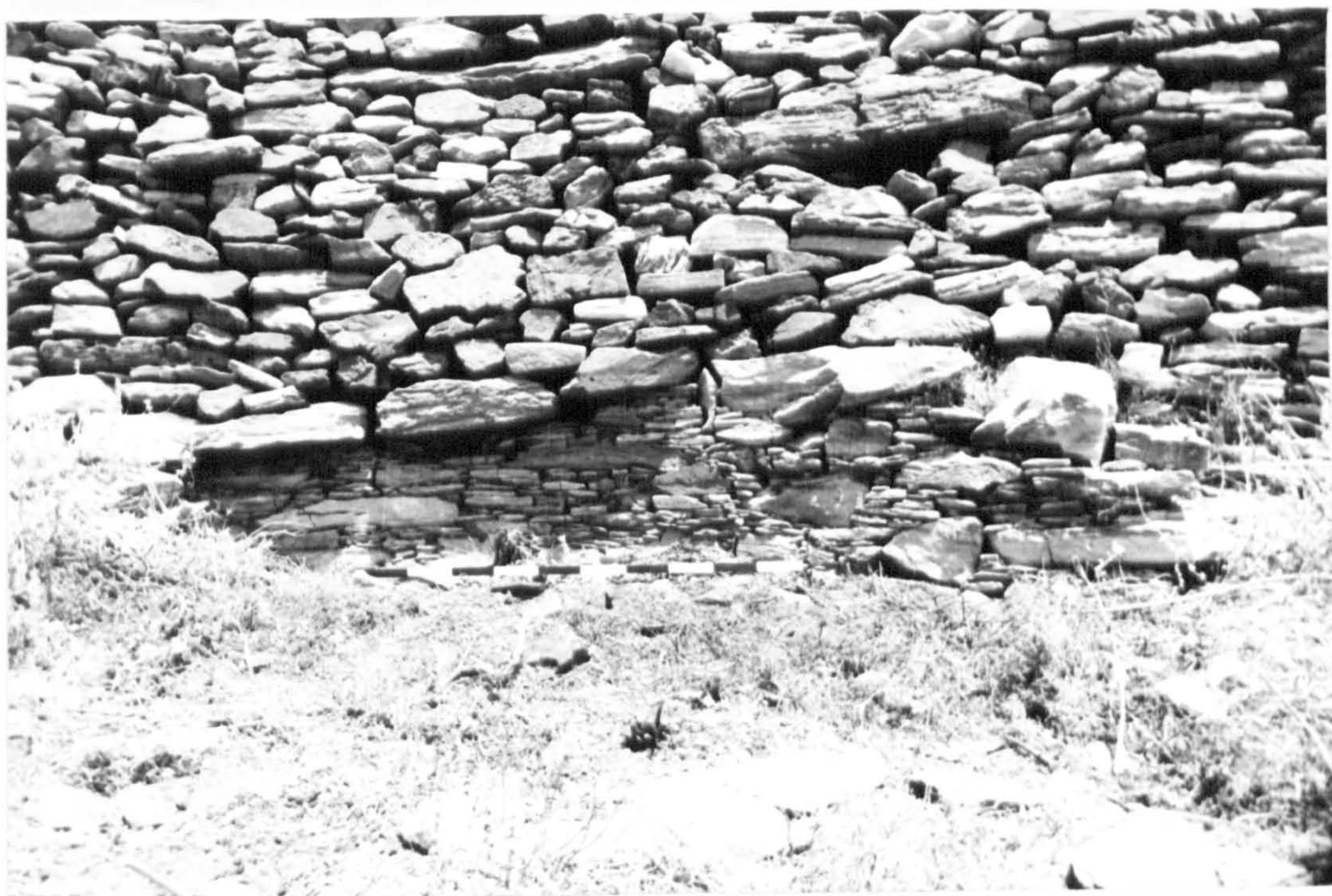
Pl. 19: TSOUKA: the interior of the tower - E side
