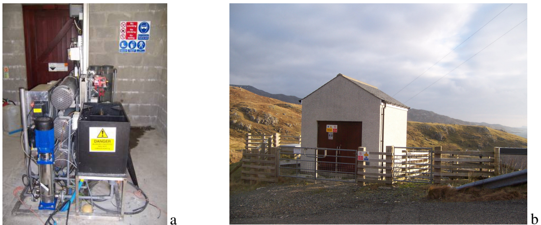
Figure A-1.5 Pictures of Plant B located on the remote western island
