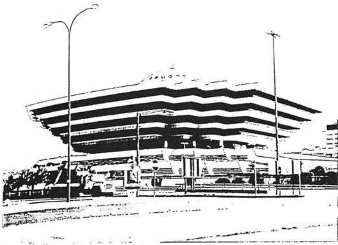
Fig. 4.19 Ministry of Interior Building
