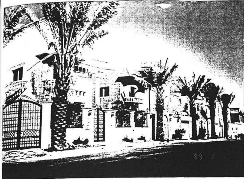
Fig. 4.25 Buildings not in harmony
