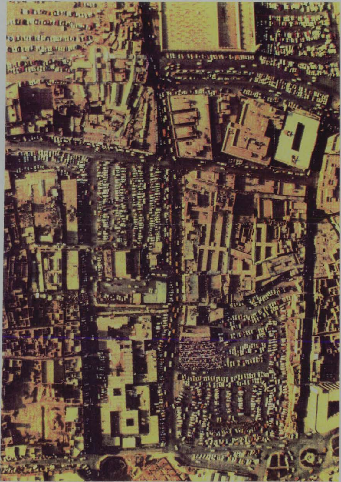
Fig.97 Aerial photograph of the JPD in 1979 showing the demand for parking areas. Source: ADA.
