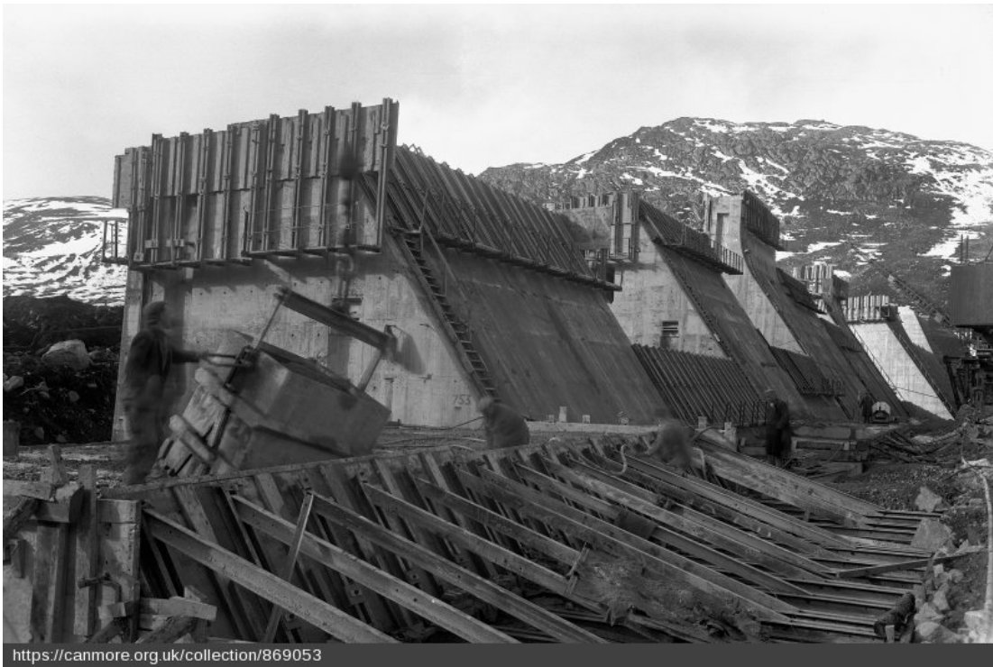
Figure 36: Mullardoch Dam, South Wing 1951, Crown Copyright HES
