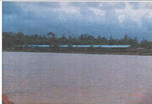
View of the front approach of the longhouse from the River Tatau
