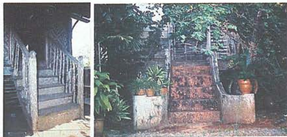
It is typical for a Malay house to have two entrances via the staircase, but this simple peasant house has also adopted a traditional Malaccan stone staircase (without the tiles) for its second entrance, adorned merely by the potted plants.
