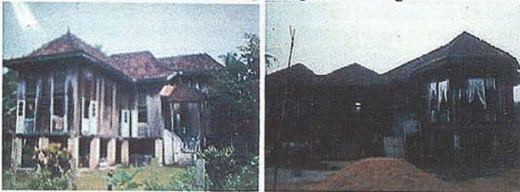
This centuries old house of Wan Embong in Terengganu is an example of a surviving timber-built house, which chose the Cengal type to create the components of the house, and which includes the leaf of the door, the archway door, the kekisi (a line of vertical panels placed in between the opening of the window), the tebar layar , the sisir angin , the walls and the tunjuk langit (Said, et al, 2002).
