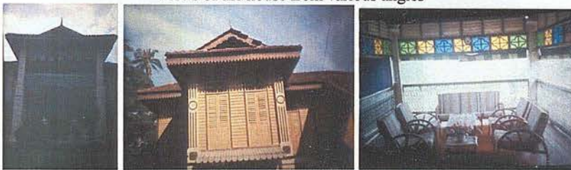
The perspectives of the 'Anjung' or entrance porch of the house and its view from the interior
