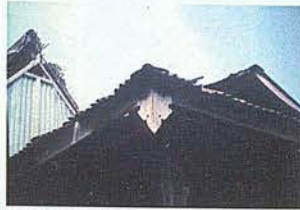
Details at the corner of the barge board below the roof.
