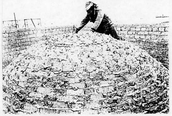
b) The finishing of the dome
