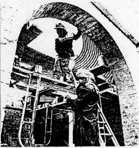
Figure 5.7: a) The RCEC during construction
