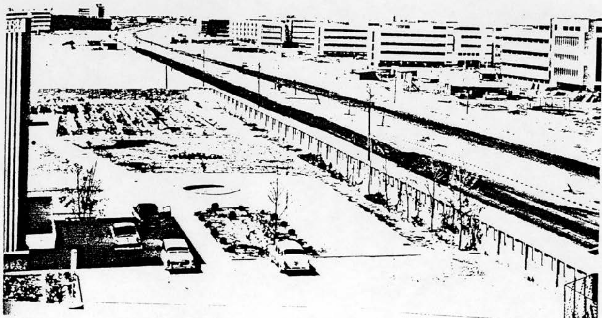
Figure 4.16: The Ministry buildings along King Abdulaziz Road. (Source: DOX-SAU-A2, 1968, p. 163.)
