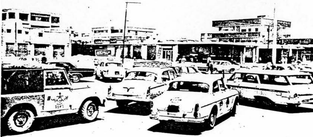
Figure 4.20: Traffic congestion and ugly buildings. (Source: DOX-SAU-A2, 1968, p. 187)
