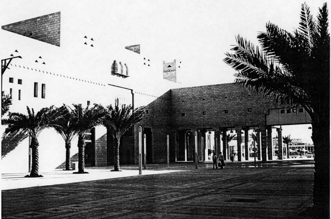
Figure 8.36: View of the Royal entrance and the bridge that connects the palace with the mosque. The photo is taken from Saḥat Alsafat looking west. (Source: Author)
