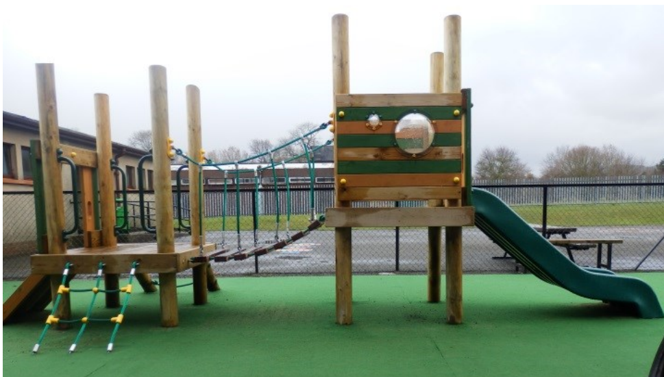
Figure 5-7: The Timber Climbing Frame
