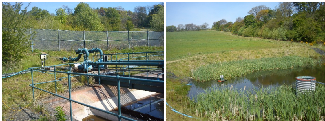
Fig. 2.4. a) Drains collecting water from the previous landfill site into the treatment plant pond, b) the collection pond.
