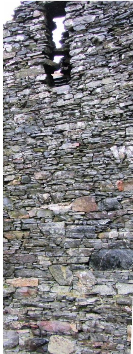
Figure 170 a & b The stacked voids at Dun Troddan, a (above) the voids over the stair entrance and b (right) the high level stacked void and the masonry beneath it.
