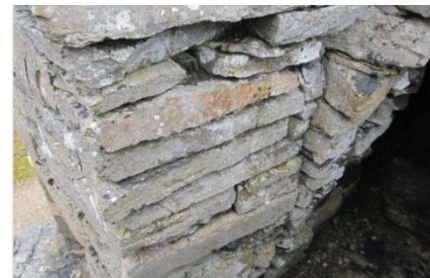
Figure 91 (above) The back of the left edge of the stairway ope. Note the building break between the vertical masonry pier and the inward leaning side wall of the gallery.
