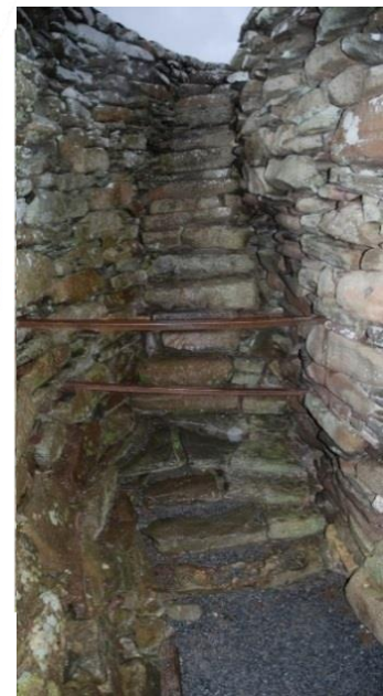
Figure 80 (above) The inner wallface of the outer wall at the secondary door. The lines indicate the more obvious fracture planes through the masonry which is clearly heavily reworked in this area.
