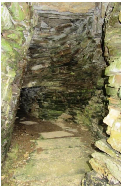
Figure 95 (left): The entrance to the pear-shaped cell from the stairfoot showing divergence of the left hand wall from the floor lintels of the original gallery.
