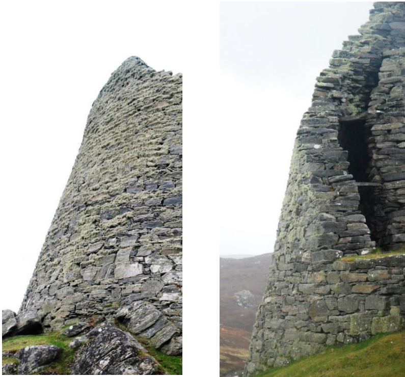
Figure 144 Comparison of outer wallface profile outwith the stacked void (left) with that at right angles to it (right). The former is kinked and faceted, the latter linear (in the vertical plane) and smoothly curved (in the horizontal).
