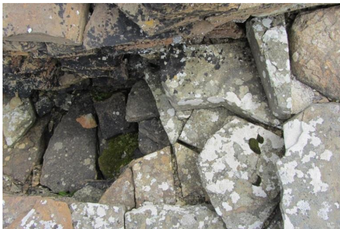
Figure 124 Slab-on-slab secondary paving inserted between gallery walls.
