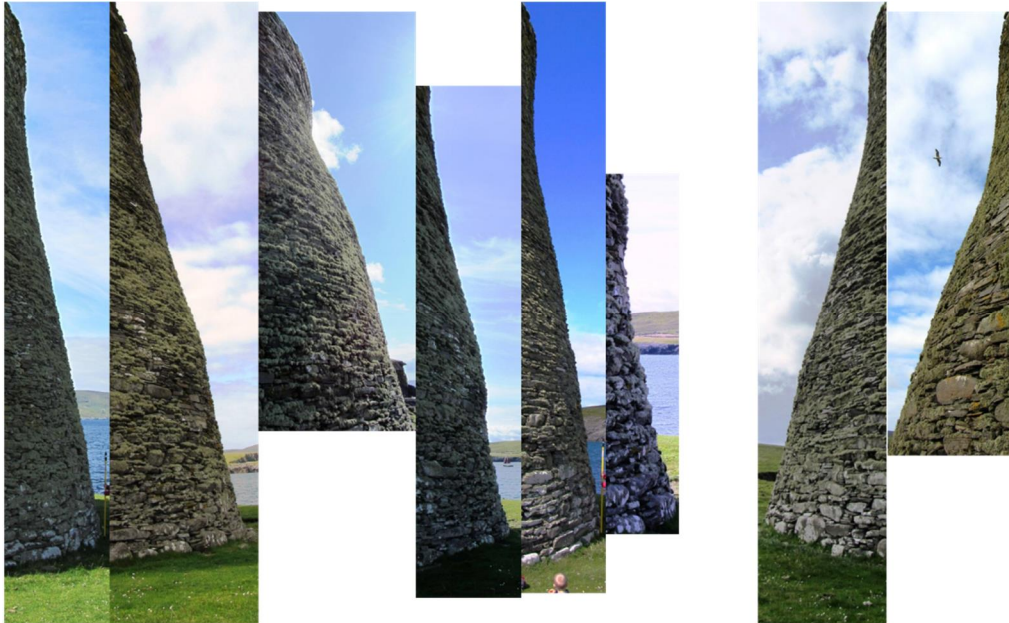
Figure 65 Outer Wall profiles at Mousa. The LHS image probably best preserves the original battered profile of the broch wall in its lower half. The various bulges and out-thrusts, in places beneath slightly overhanging upper part is most probably Viking in date. (These images are only approximately correctly aligned for height relative to each other).
