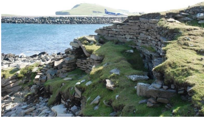
Figure 175 Broch at East Shore, Pool of Virkie, Shetland. The inner wall and its scarcement are visible on the right and tumble and collapse near the centre fall away to the foreshore sloping down some 3 m below, to the left. The LHS of the broch had been built on unconsolidated material
