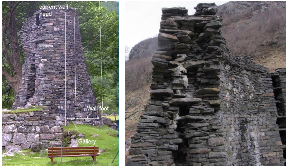
Figure 35 Dun Telve, Glenelg is illustrated here to show that the outer and inner walls converge with height and meet just below the wallhead. The high scarcement is visible in the right hand image and it is generally speculated that this lies at the wall convergence level and perhaps 1 m or so below the final wallhead. The weeping lime salts probably result from relatively recent conservation, some of the stones of which can be seen just right of the excrecence, supporting the view that the stones filling the intramural space above that level are as originally built
