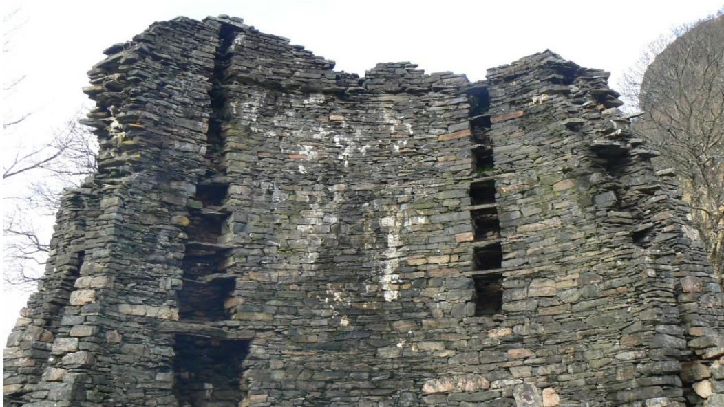
Figure 154 The inner wallface, like the surviving outer wallface is extremely well built and has preserved in relatively good condition throughout. The quality of the build is indicative of Iron Age construction rather than overactive modern restorative conservation.
