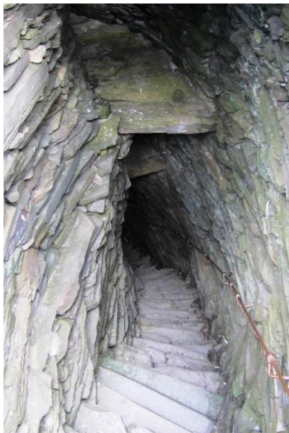
Figure 59 (left) View down the helical stairway, revealing two gallery floors. Note the several adjustments to the curvature and location of the left hand wall, i.e. the wall abutting the interior of the broch. This wallface has been stepped back from the stairwell in three stages and follows a recurved footprint in the uppermost. It is probable that this is associated with the secondary insertion of the helical stairs.
