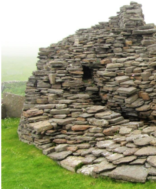
Figure 116 (left) The West end of the breach in the outer wall. Note how the entrance masonry, visible top left, is horizontally set above the tilted masonry of the edges of the breach in the wall
