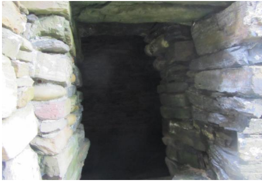
Figure 110 The short access passage to the LHS Guardcell. Note the building join in its right hand side wall.
