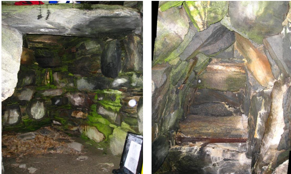
Figure 169 the stairfoot cell, (left) viewed from the entrance and (right) its roofing.
