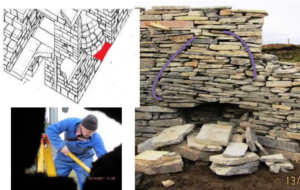
Figure 31 The sketch (top left) shows the attenuated footprint of the inner wall, shaded red. Any settlement into this footprint would lever the inner wall inwards from the stepped stones of the corbelled guardcell. This was simulated in a 1:1 model of the Clachtoll entrance and forced into failure. However, the stones above simply arched over the breach (curved purple lines). The breach was pushed through the guardcell wall (bottom left) with no further failure of the wall masonry
