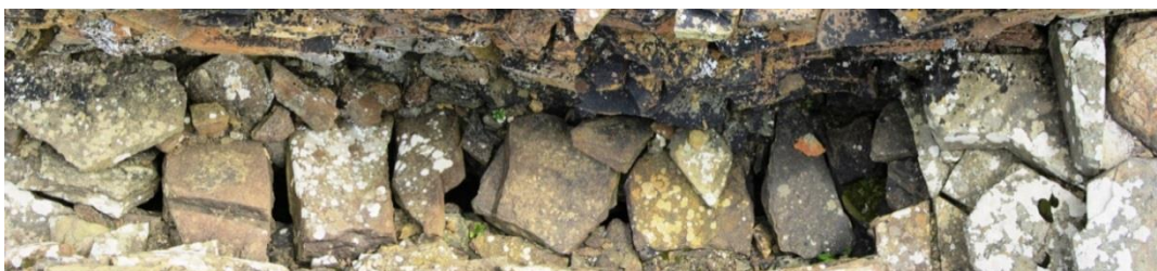
Figure 123 (above) Original roof lintels of the ground gallery, many broken and displaced, under levelling deposit of slabs and upper slab pavement (on far right).
