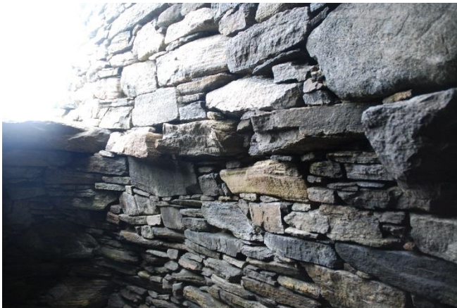
Figure 150 (left) The stumps of broken roof lintels of the 9 o'clock cell visible in the inner wallface of the outer wall.
