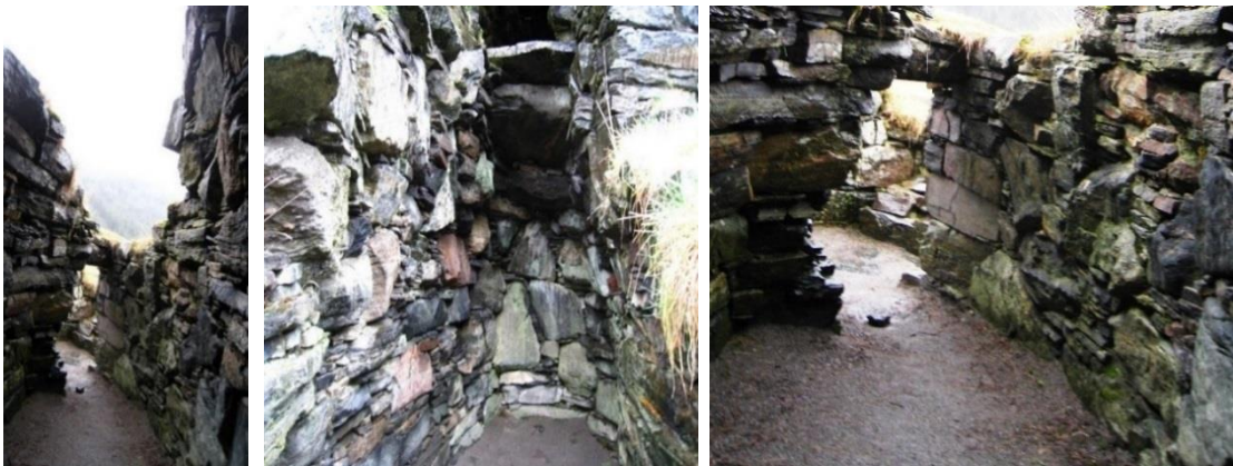
Figure 168 a & b The LHS guardcell, (a, left) looking towards the entrance and (b, middle) back of cell and (c right) The guardcell entrance.
