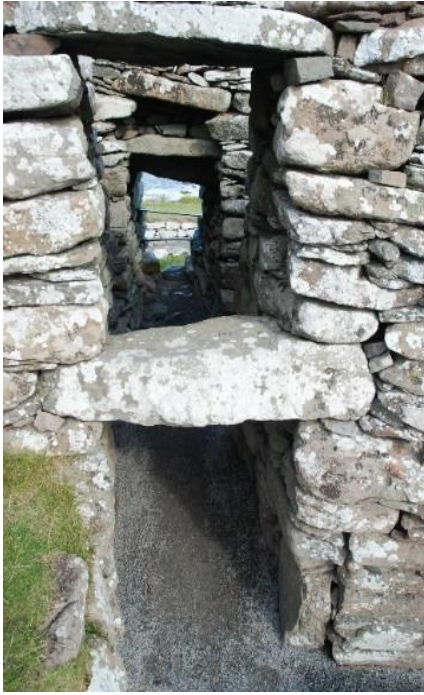
Figure 78 (left) The reuse of a stacked void, probably the original stair landing stacked void, to form an entranceway through the inner wall. The entranceway passage cut through the wallhead for about 600 mm and crossed the first level gallery void to exit the broch by a new ope slapped-through the outer walling of the monument.
