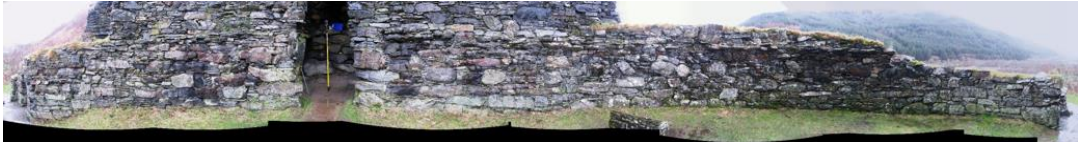
Figure 167 The inner wallface at Dun Troddan illustrating the scarcement level.
