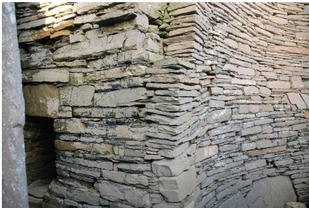
Figure 111 The ILW at the entrance passage (LHS) The deep concavity of the wall is indicated by the sweep of the masonry lines. The stumps of the original passage lintels are visible top left of the image where the innermost lintel, now lost may have lain in a scarcement at this level. It is probable that the broch wall was substantially rebuilt above this level.
