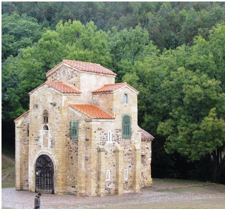
Figure 14 San Miguel de Lillo, Naranco; surviving fragment. The emergent Asturian cruciform is represented in this church only in the projection of transepts above the line of the side aisles on the exterior. That line was continued into a much larger nave, now lost but represented in cobbling behind the church (visible bottom right in this picture).
