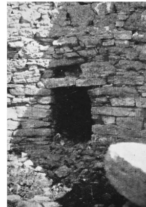
Figure 135 (above) Sealed voids of relieving structures over cell entrances: the blue rectangles mark the void locations in the thumbnails above the main images.
