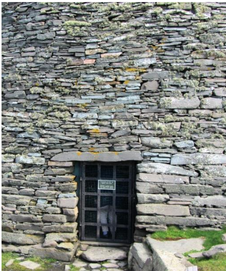
Figure 63 (left) The outer wallface above the current entrance at Mousa. The edges of the inserted masonry are indicated by a proliferation of small slabs and an extensive rispains joint on the right.
