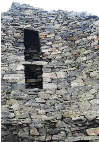
Figure 143 The relict stacked void fragment above the scarcement at Dun Carloway.
