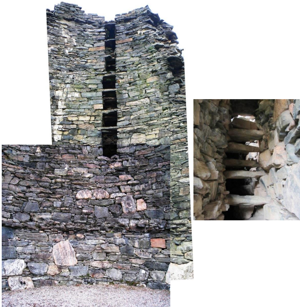
Figure 162 a Dun Telve, (left) the stacked void at the 8 o'clock position in the inner wallface at Dun Telve. b (right) The inter-mural struts that propped the edges of the now closed-off stacked void segments below the surviving elements.
