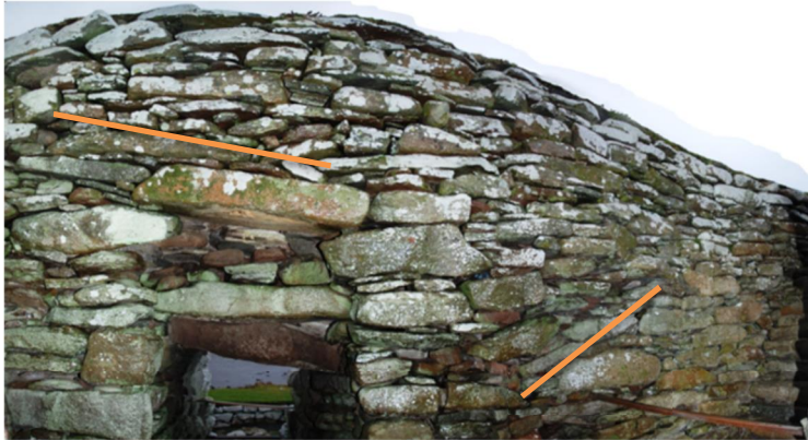
Figure 80 (above) The inner wallface of the outer wall at the secondary door. The lines indicate the more obvious fracture planes through the masonry which is clearly heavily reworked in this area.
