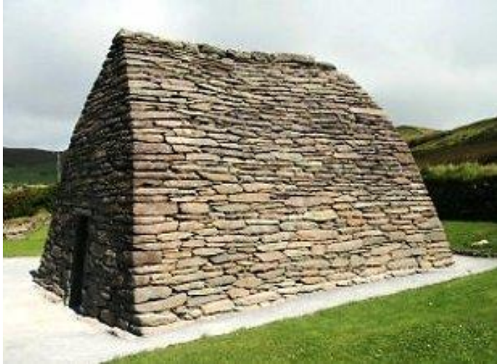
Figure 6 Gallarus oratory, Dingle, Ireland. A corbelled oratory which may have been built with mortar. Its date is disputed but may lie in the range 800 to 1200 AD although some scholars suggest a much earlier, even pre-Patrician dates.
