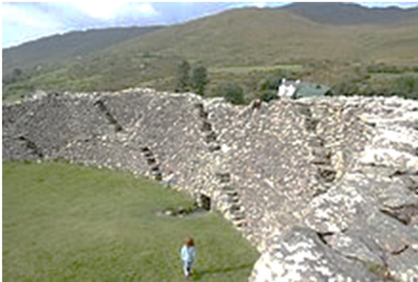
Figure 51 The Irish stone fort at Staigue, Co. Kerry, comprises a large curtain wall with characteristic X-shaped stairways built into the internal wallface.
