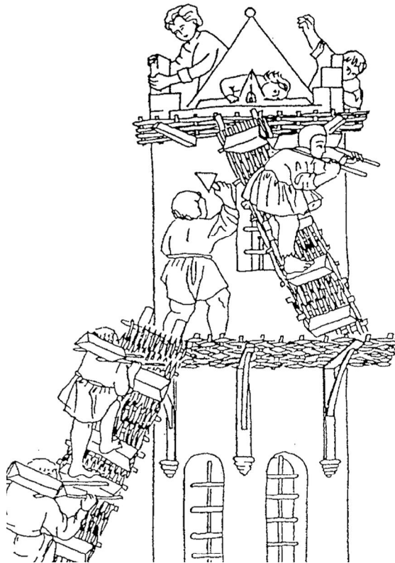
Figure 33 In this illustration dating to c. AD 1300 the long ladder/ramps have been stiffened behind by stronger poles, but otherwise the ramp-ladder and the hanging scaffoldings are clearly of wattle work. Note also, the little figure at the wallhead levelling with a plumb-level. Save only for the use of mortar – evidenced by the trowel – there is nothing in this illustration that could not be encountered in the Scottish Iron Age. (after the British Museum’s Egerton manuscript, as reproduced in Binding 2004, 87, his Figure 268: creative commons ©).
