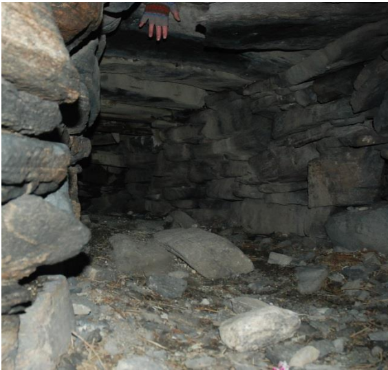
Figure 149 A view along the intramural void entered from beneath the blocking wallface. The hand visible top left has been inserted from the landing element of the stairway.
