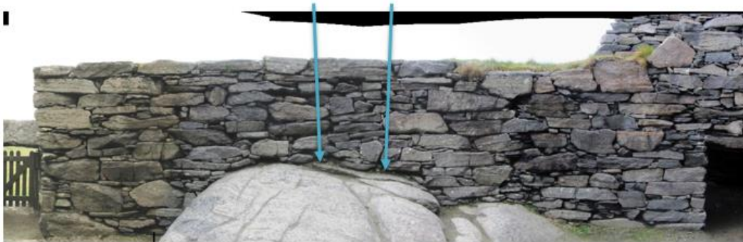
Figure 134 Inner wallface elevation panorama (2a) with detail of possible cell entrance at the 7-8 o'clock position (2b).
