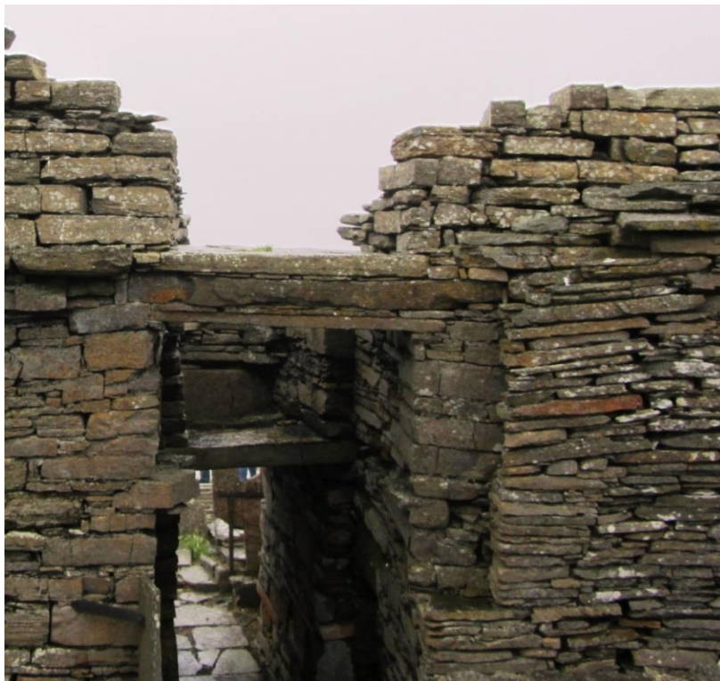
Figure 108 View of the entrance passage from inside the broch.
