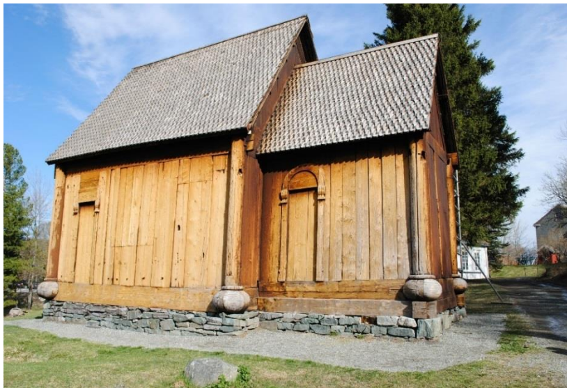
Figure 8 The simple stave built church of Haltdalen, Norway. Note that the structure is supported on a stub wall, which is all that would survive the decomposition of the church.
