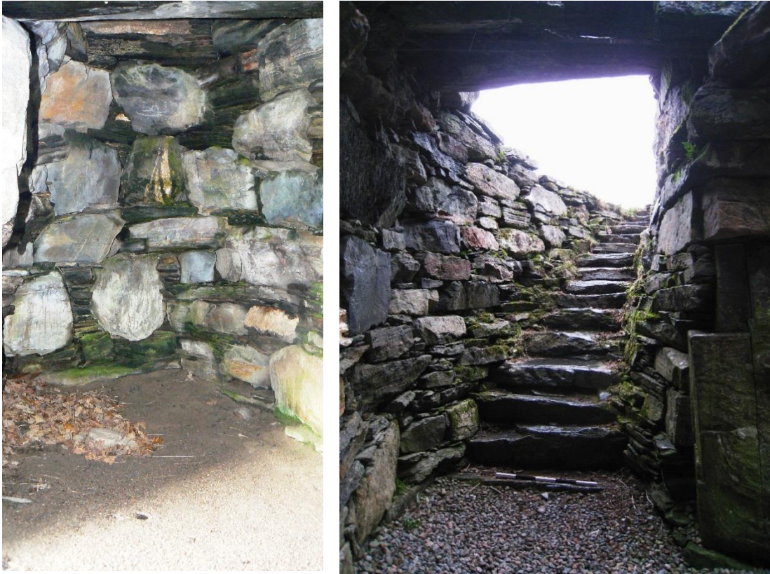
Figure 161 a & b. Dun Telve, the stairfoot. The counter stairfoot cell (left) and the ground floor stairway (right).
