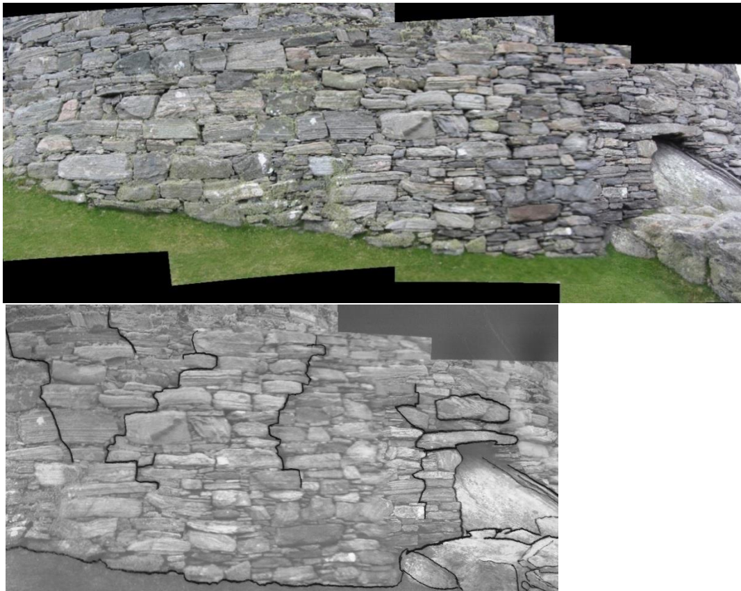
Figure 139 (above) The outer wallface of Dun Carloway on the southwest side (entrance just off the image to the left). A proliferation of fabric replacements is visible above and left of the bridging slabs over the bedrock. (below) A field sketch shows divisions between apparently different masonry masses
