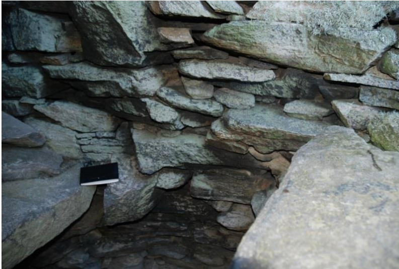
Figure 141 (left) Tusings from broken lintels of the 3 o'clock cell. The lintel visible bottom right is a new insertion.
