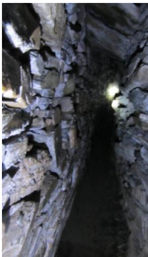
Figure 87 View along the ground gallery from the LHS guardcell
