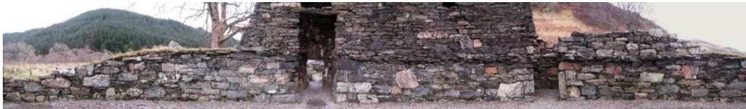
Figure 156 The low level scarcement elements in this scarcement. The higher scarcement is preserved in the less than a third of the circuit that survives to near full height. It should be noted that the stacked voids at the entrance and the 8 o'clock position continue above the level of the upper scarcement.
