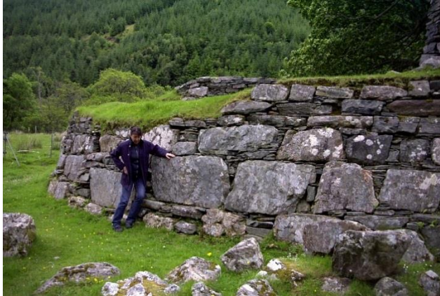
Figure 153 The outer wallface at ground level includes many very large stone blocks and slabs.
