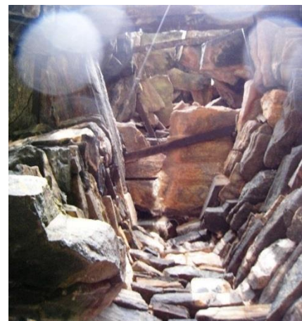
Figure 163 The entrance stacked void (left). It is clear that several transverse struts have been lost and many of the surviving struts are broken. The image below illustrates the poor condition of many of the remaining struts in this view up through the entrance stacked void.
