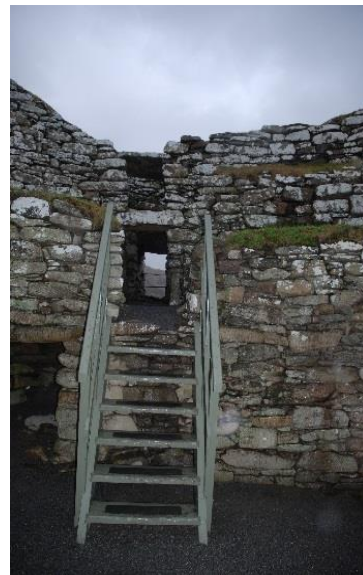
Figure 76 Cell A at Clickhimin (RCAHMS nomenclature). The garth-side corbelled shell is propped against the near vertical outer wall fragment and lintelled over for closure.
