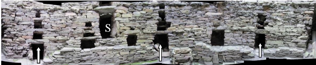
Figure 66 The internal wall foot at Mousa. The broch entrance appears at both ends of this panorama. Short stacked voids are positioned over the entrance lintels of the wall cells and some aumbries. The wall between the entrance, on the left in this image, and the stair access ‘S’ seems extensively rebuilt.
