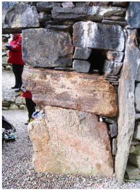
Figure 160 (left) The bar receiver and jambstone, adjacent to the guardcell entrance.
