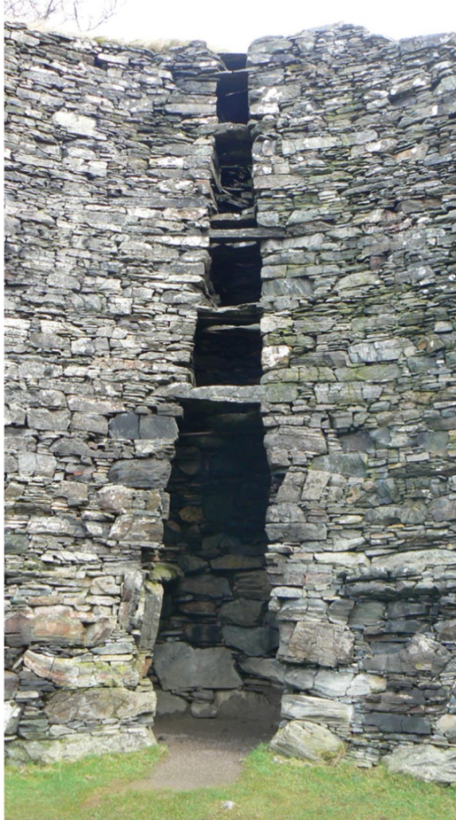
Figure 170 a & b The stacked voids at Dun Troddan, a (above) the voids over the stair entrance and b (right) the high level stacked void and the masonry beneath it.
