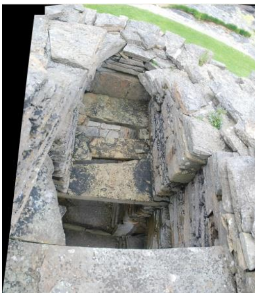
Figure 112 The supra-entrance cell viewed from the upper lintel table; note tussing (on left) of a lost innermost upper lintel which had extended this lintel table to the line of the doorjamb.
