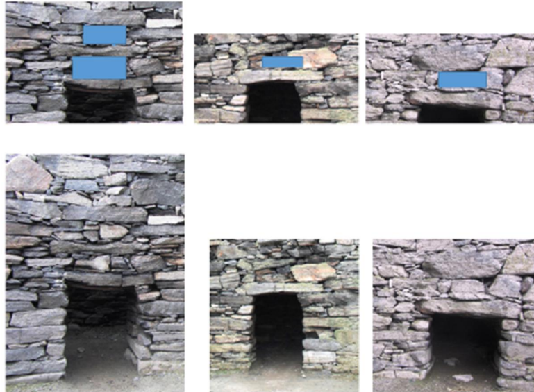
Figure 135 (above) Sealed voids of relieving structures over cell entrances: the blue rectangles mark the void locations in the thumbnails above the main images.
