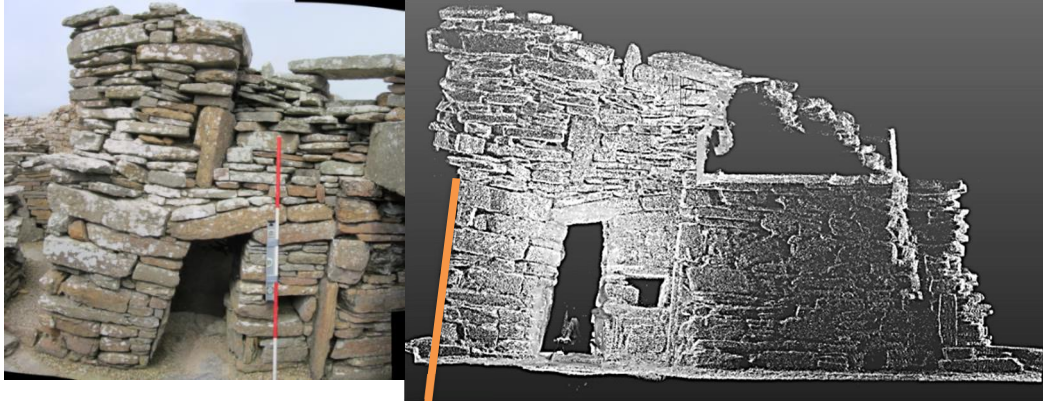
Figure 122 The photographic panorama of the entrance area of the broch (left) exaggerates some of its proportions, but the laser scan (right) is metrically precise.
