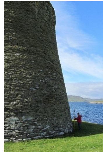
Figure 64 (right) Profile on the north east of the monument is steeply battered and linear in section to about mid-height above which it becomes vertical, in two stages.
