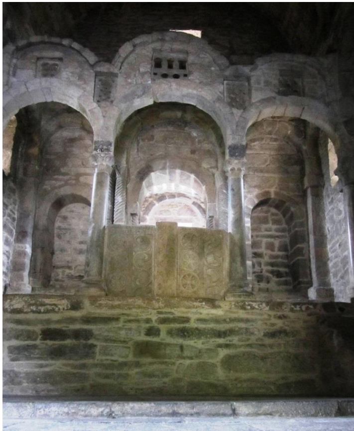
Figure 15 Sancta Cristina de Lena. The raised chancel with iconostasis-like arrangement of decorated slabs between pillars (above). The apparent depth of the chancel area is an optical illusion; it is less than 1.5 m deep. The narrow access steps are out of shot to the right and left in this image (see plan below).
