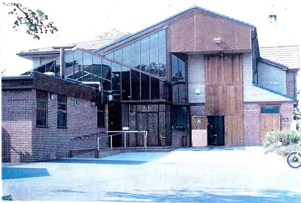
FIGURE 4 View of the present day Veterinary Investigation Centre at Sutton Bonington. The post-mortem room is to the right and the incinerator lies behind.
