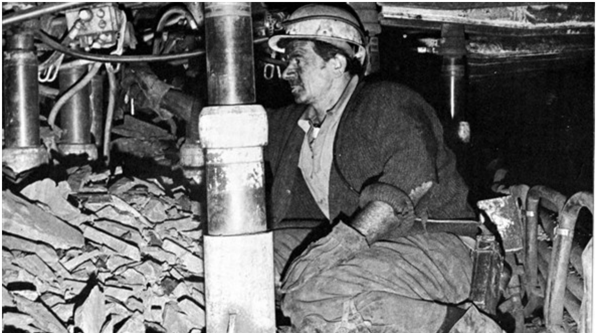
Upper left: cover for NCB brochure for Mansfield Colliery. Upper right: schematic of roadways and longwall panels at Mansfield Colliery. Lower: A miner advancing hydraulic chocks at Mansfield colliery circa ~1970's. The normal working height of the seams was ~4 ft (1.2 m). Photos © NCB and www.ourmansfieldandarea.co.uk , and reproduced here with kind permission.
