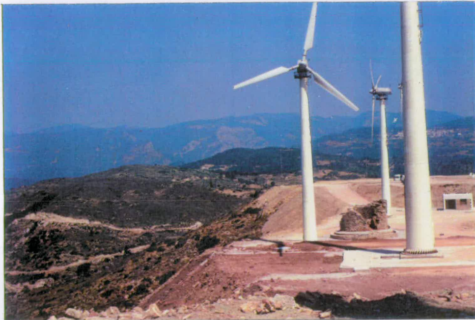
Figure 4.2.1(i) Vestas WM19S wind turbines on Samos Island, Greece.
