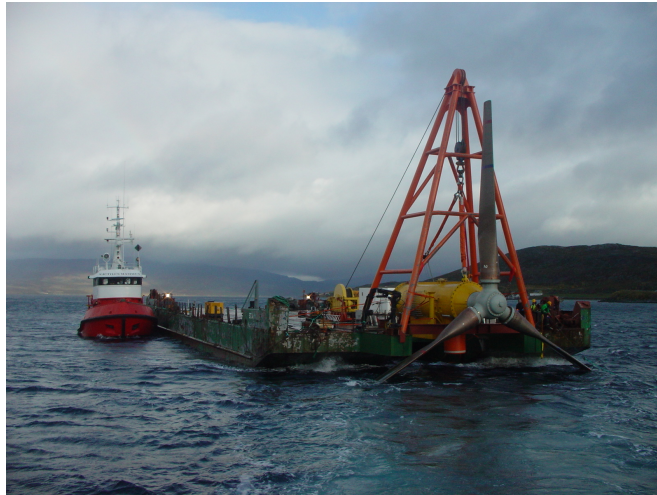
Figure 2.2: The Hammerfest HS300 during installation (Andritz Hydro Hammerfest, 2012).
