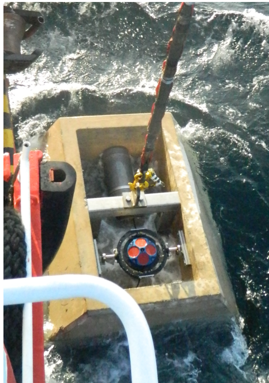
Figure 3.10: A DBDP mounted in a gimbal on a concrete gravity base during deployment.
