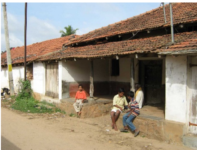
Figure 7. Jagali transition. This transition space was and is used for the most part of the day for different activities. This climate-responsive space would have been in the shade for most of the day
