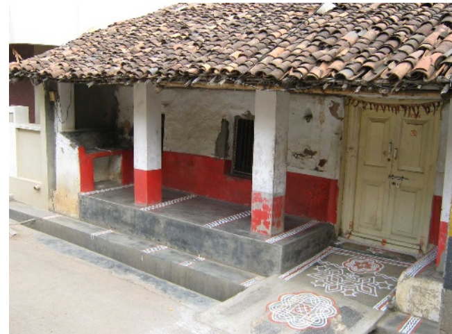
Figure 9. External space. This view of the jagali clearly shows the way the house engages with the surroundings. This part was and is used for most of the day. It also reflects the use of locally available material and culture
