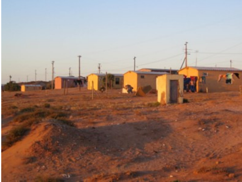
Picture showing housing and electricity infrastructure in Papendorp.
