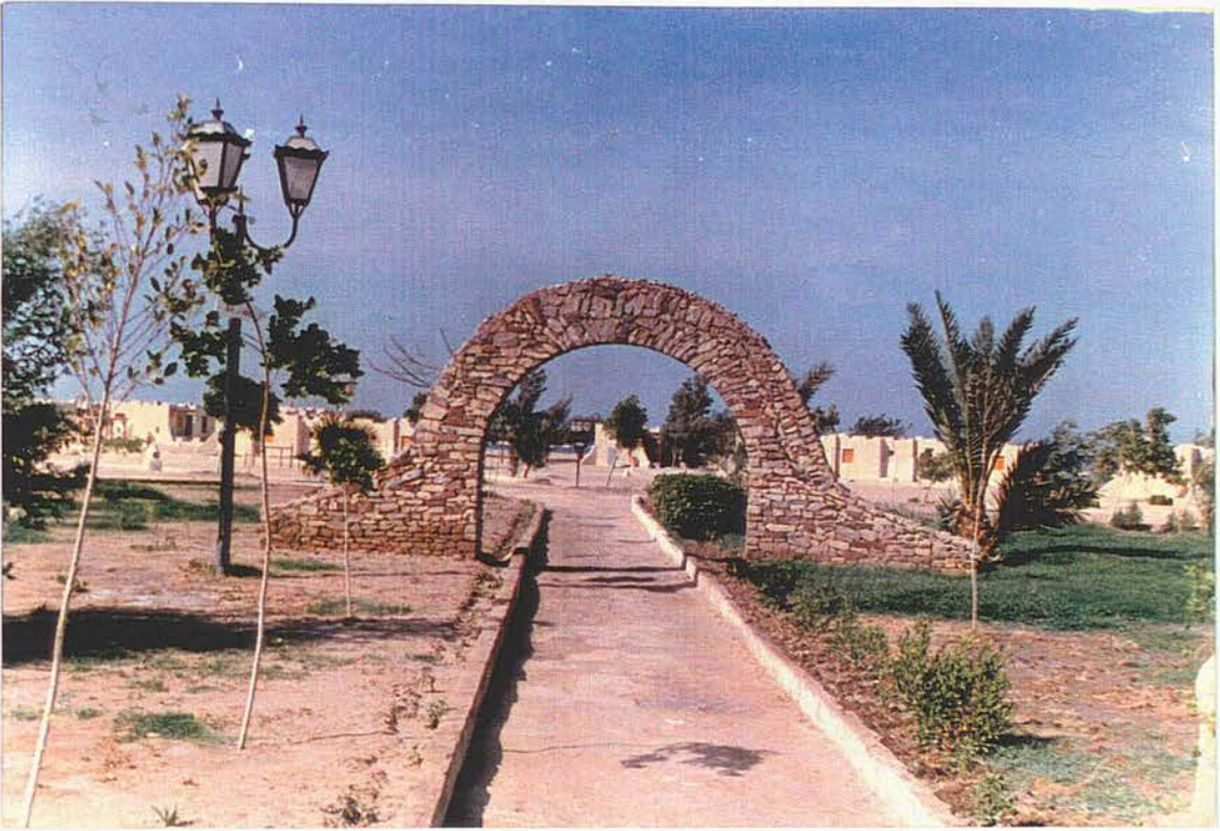
Figure 6.61: Poor attempt in the use of design elements, still no shade is provided. (Magaweesh Resort)
