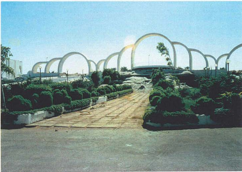
Figure 6.60: Construction work is poor, and the design has no clear purpose. (Arabia Resort)
