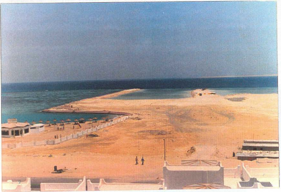
Figure 6.15: Showing the land fill reaching the deep coral slope (the dark blue line in the Photograph) in 'Merit' as in 'Arabia' resorts. (7/1992)
