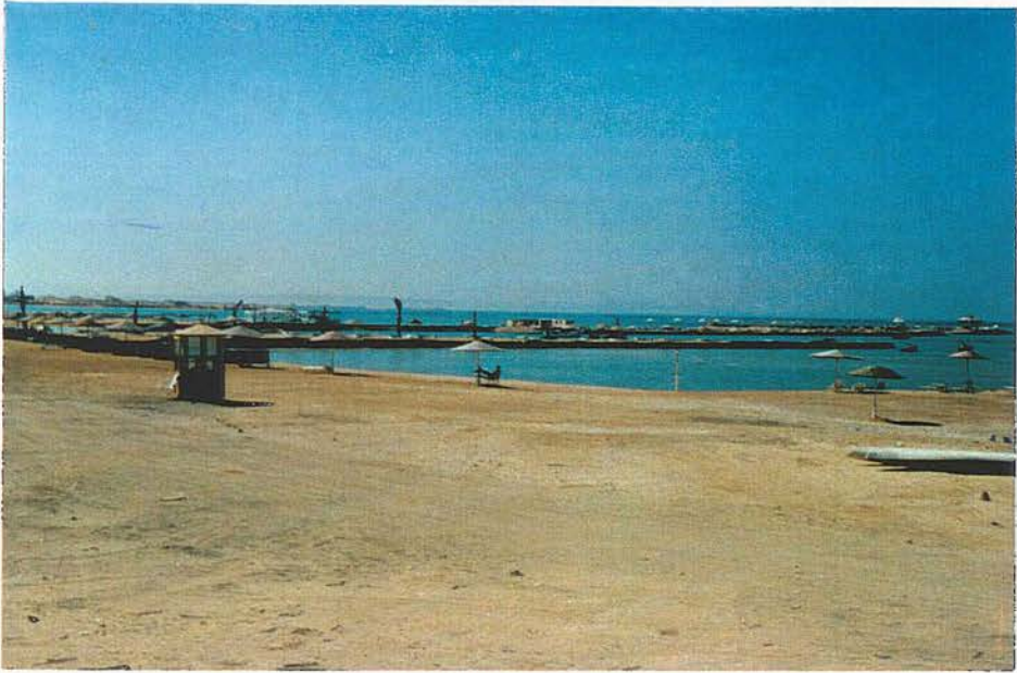
Figure 6.16: The 'Three Corners Resort', showing the land filling in the form of pedestrian walks. (8/1993)
