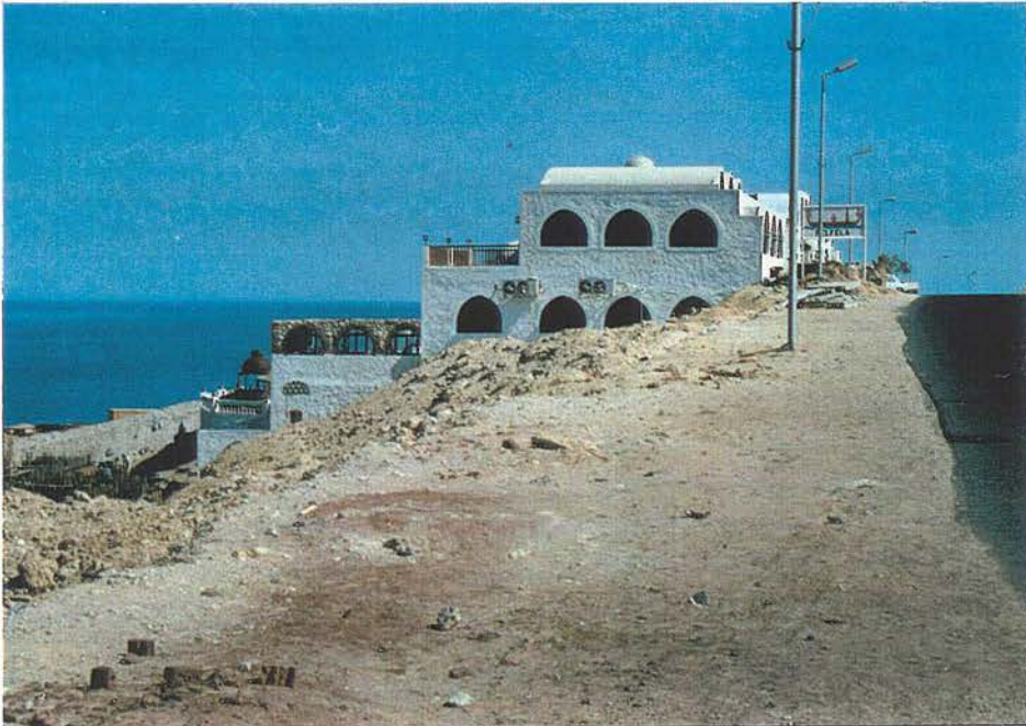
Figure 6.24: 'Felfela' restaurant, photographed in August 1993, showing the seaward extension of the building (on new land filling).
