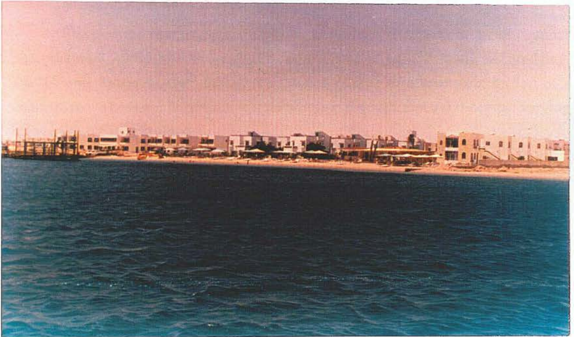
Figure 6.33: 'Mashrabya' resort. The off-shore restaurant is under construction at left. (7/1992)
