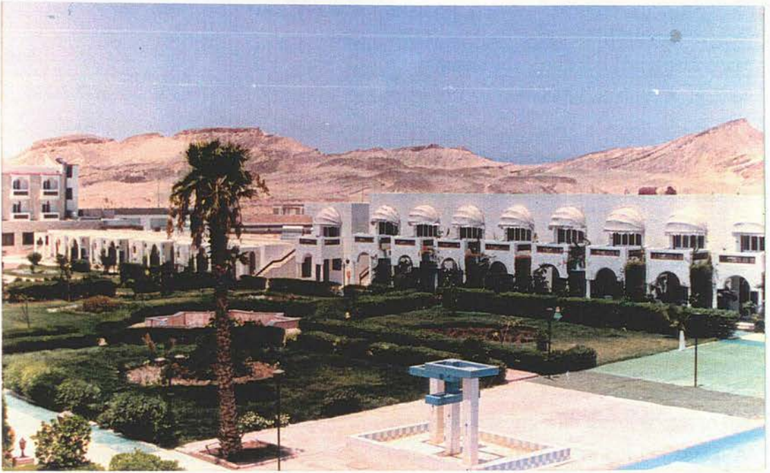
Figure 6.70: Courtyard treatment is too grand for the scale of the surrounding buildings. (Mashrabya Resort 7/1992)
