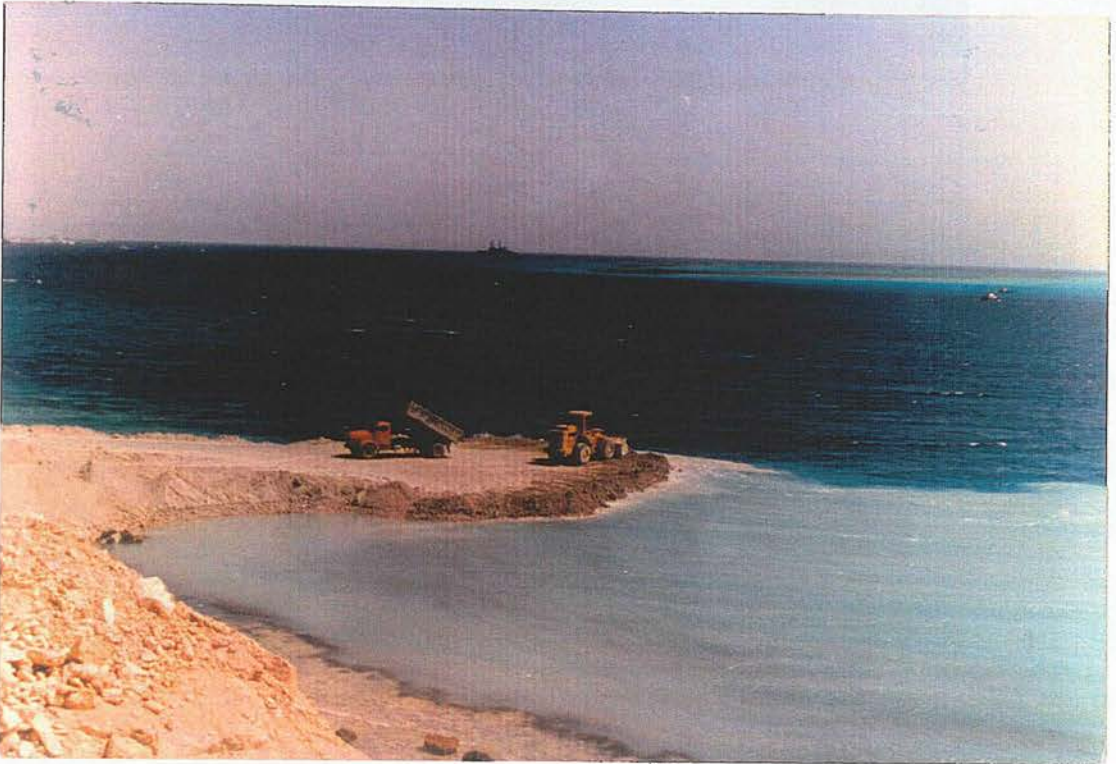
Figure 6.25: Showing the gross siltation of the water as a result of the land fill process. (Felfela Site 7/1992)
