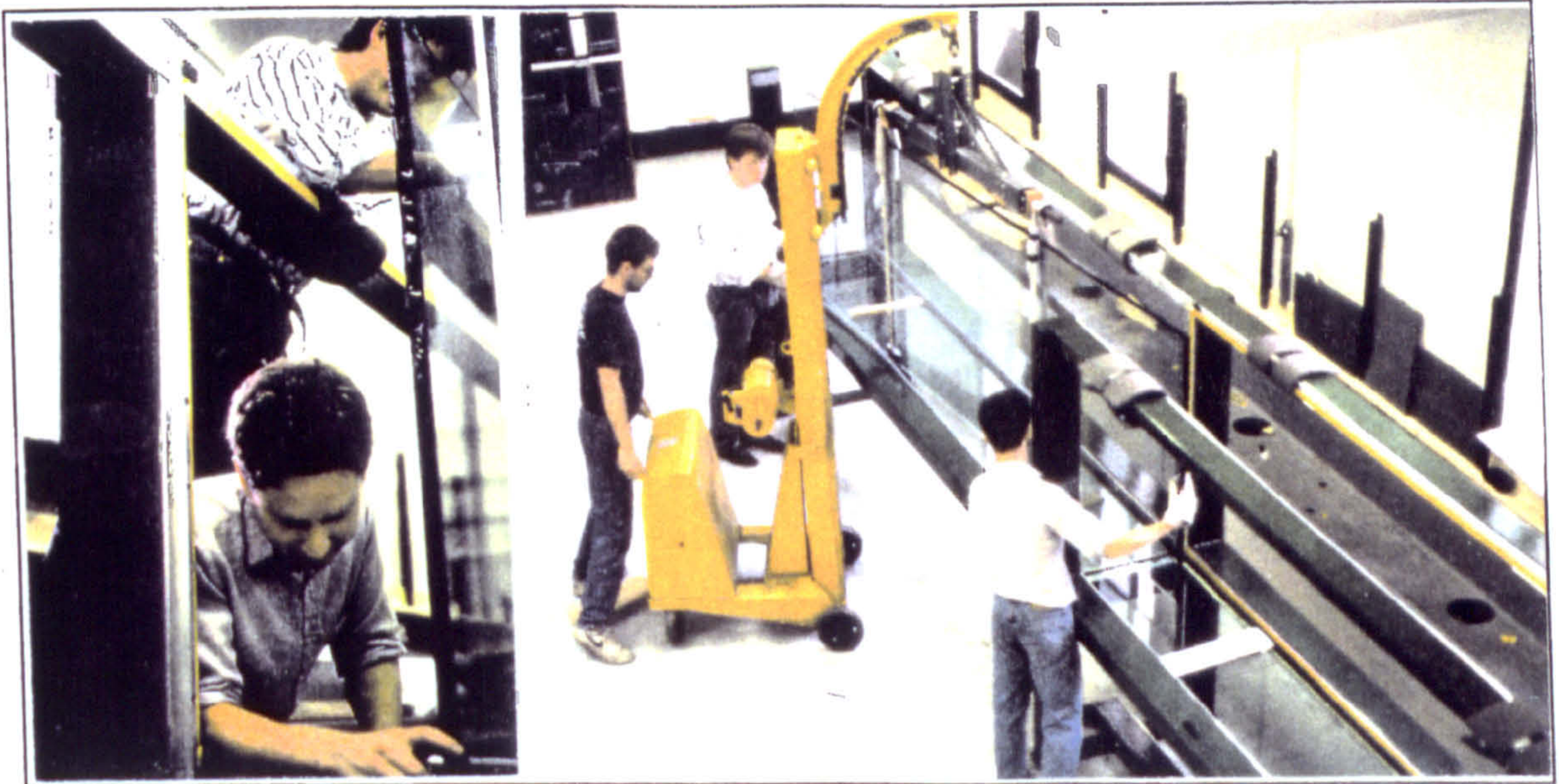
Figure 3.6: Construction of the wave flume
