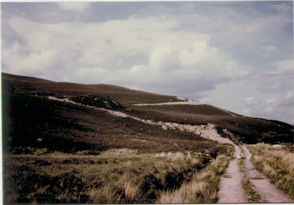
Plate 3.1 Poorly aligned actively eroding track in Glen Einich, Cairngorms NNR. Constructed circa 1960, upgraded circa 1975.
