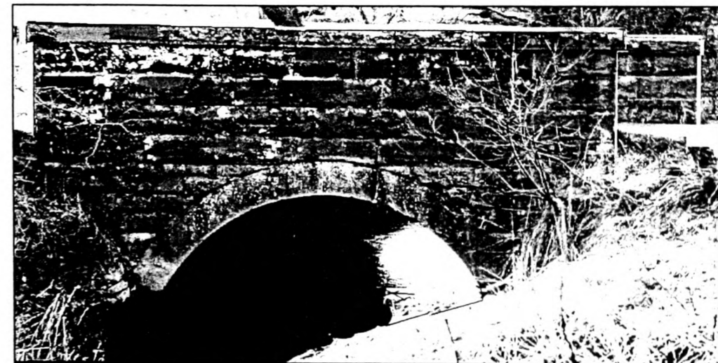
Figure 7. Kilbucho Bridge: downstream view.
