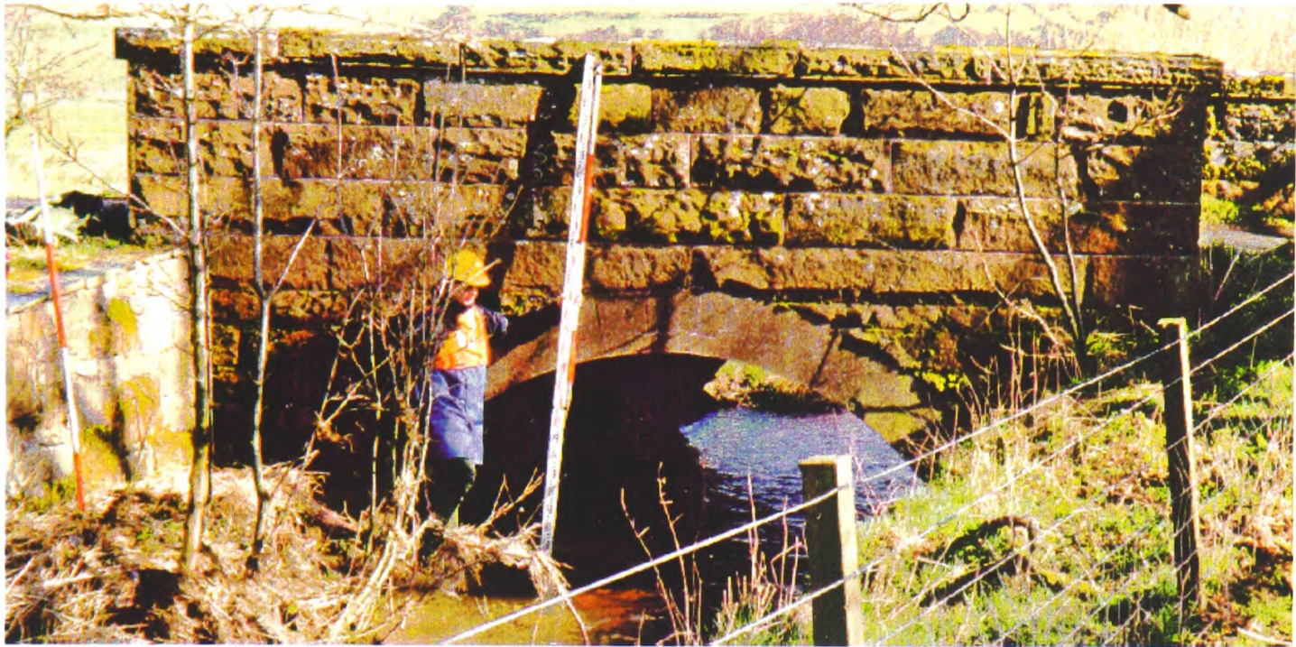
a) Downstream view.
