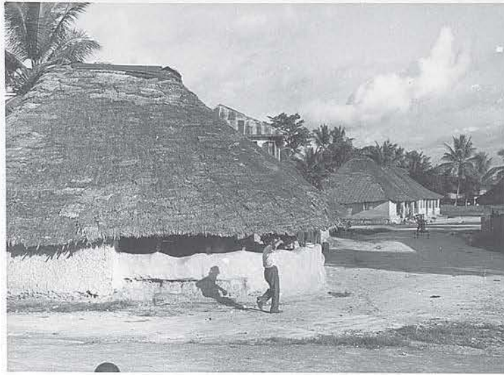
Plate 6. Old town; one of the oldest houses in Lunsar
