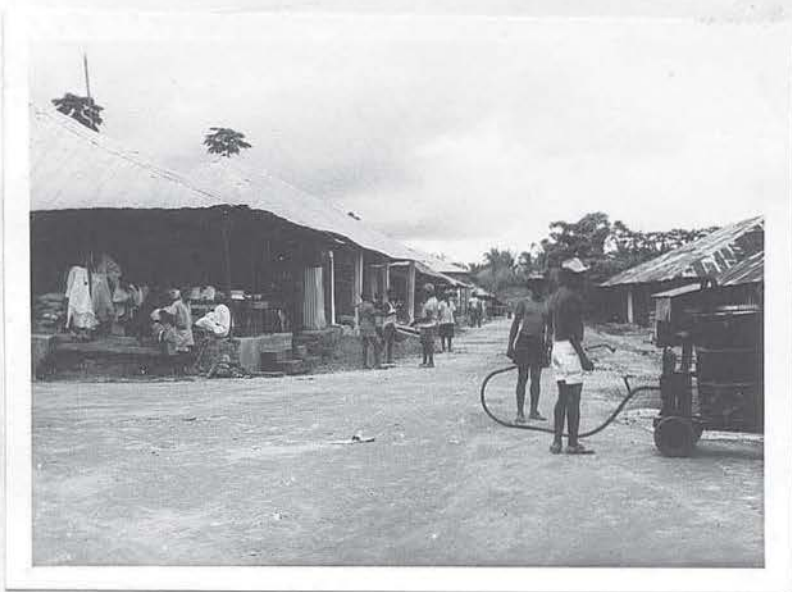
Plate 12. Tar spraying the main street. On the left are a group of Fulbe watching.
