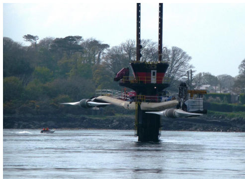
Figure 1.1: MCT SeaGen 1.2 MW twin rotor device (with platform raised for maintenance), Strangford Lough, Northern Ireland. Photo by taken by author, 03.2014
