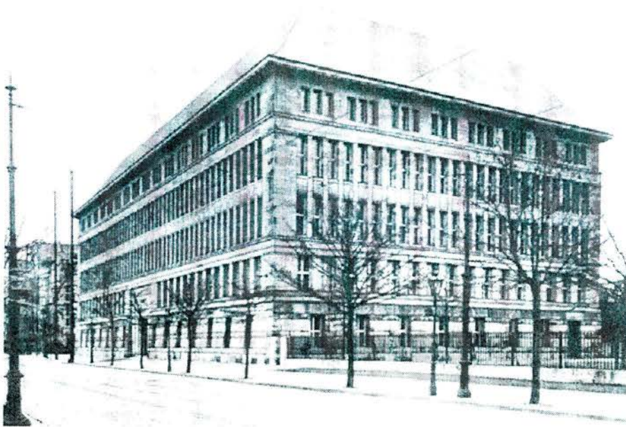
Figure 57 Peter Behrens, Mannesmann Department Store, Düsseldorf, 1911-12. (Stanford Anderson, Peter Behrens and a New Architecture for the Twentieth Century , 2000, 195)
