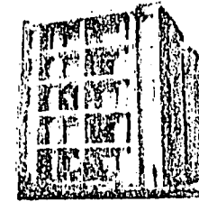
India 1976 5 storey wall thickness: 23 cms
