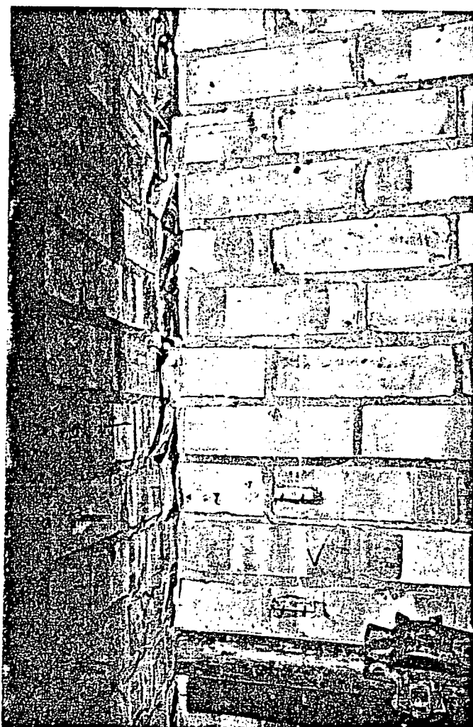
Figure 2. Showing the cracks at the intersection of main wall and return.
