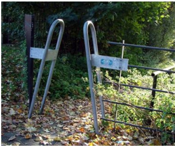
Figure 5.1 – motorcycle inhibitors. These are used as a deterrent for illegal motorcycle access to public green space.
