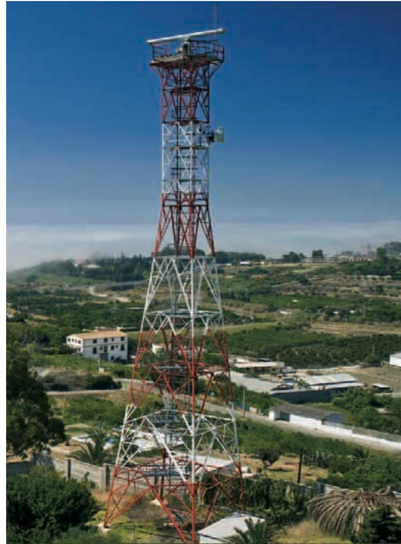
Figure 19 shows the SIVE radar tower protecting the landscape from what might lurk in the bank of encroaching fog. Original caption reads: “A bank of fog covering the coast of Estepona (Málaga) straight in front of a sensor station” (Guardia Civil 2008, p111). Published with the permission of the Guardia Civil.
