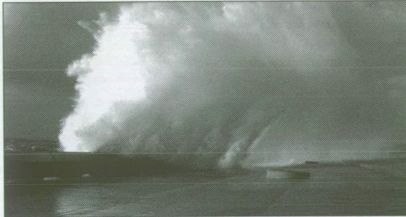
Figure 3: Violent wave overtopping at Samphire Hoe (Photograph courtesy of Eurotunnel and the White Cliffs Countryside Project)
