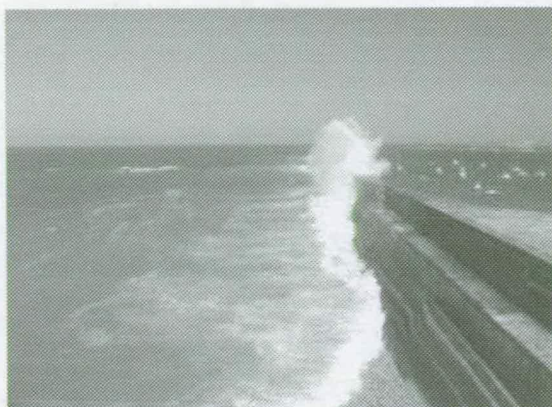
Figure 1: A broken wave overtopping the Admiralty Breakwater, Alderney (photo courtesy Gerald Müller / EPSRC BWIMCOST project).
