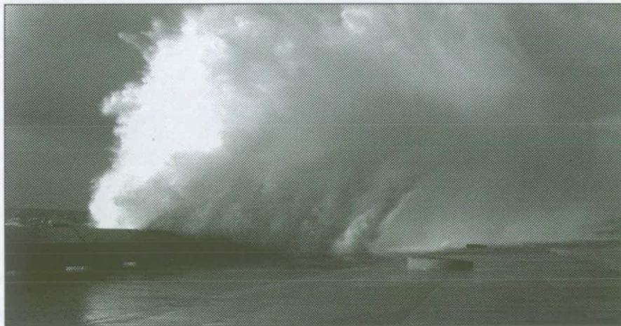
Figure 3: Violent wave overtopping at Samphire Hoe (Photograph courtesy of Eurotunnel and the White Cliffs Countryside Project)
