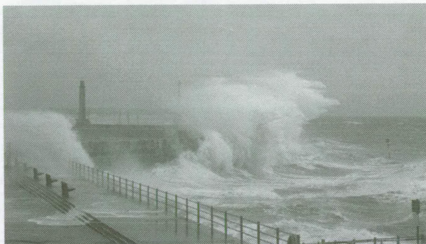
Figure 1: Overtopping event at a corner (Margate).
