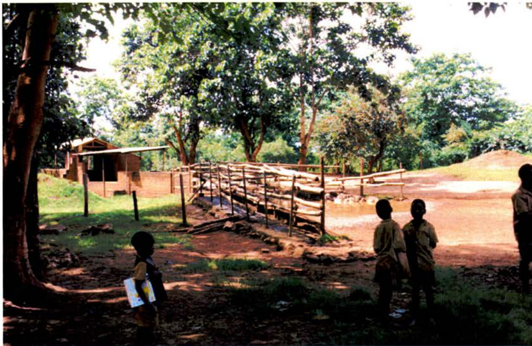
Photograph 1.6 Dixon dip tank and collecting pens. This tank was well constructed. Roofing to keep rainwater out of the tank can be seen. Erosion around the tank due to repeated gathering of cattle is also visible.
