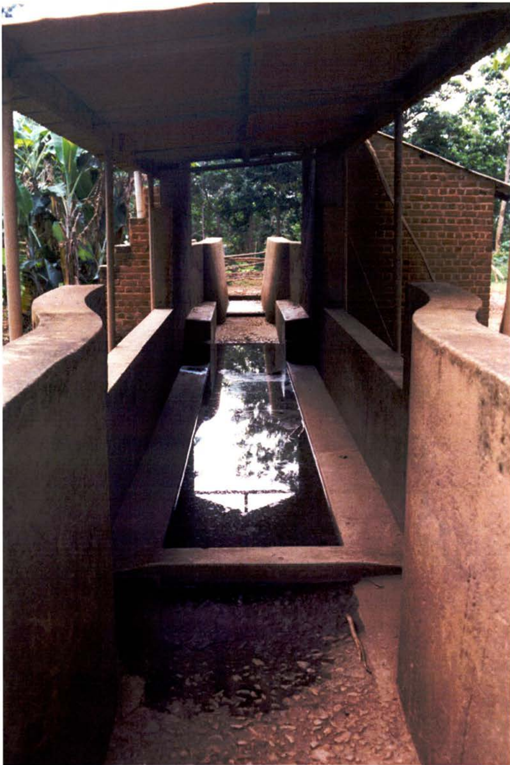
Photograph 1.7 Dip tank. Cattle exit tank in the foreground of the picture. The chemical store is situated near the entrance to the tank on the right of the picture.
