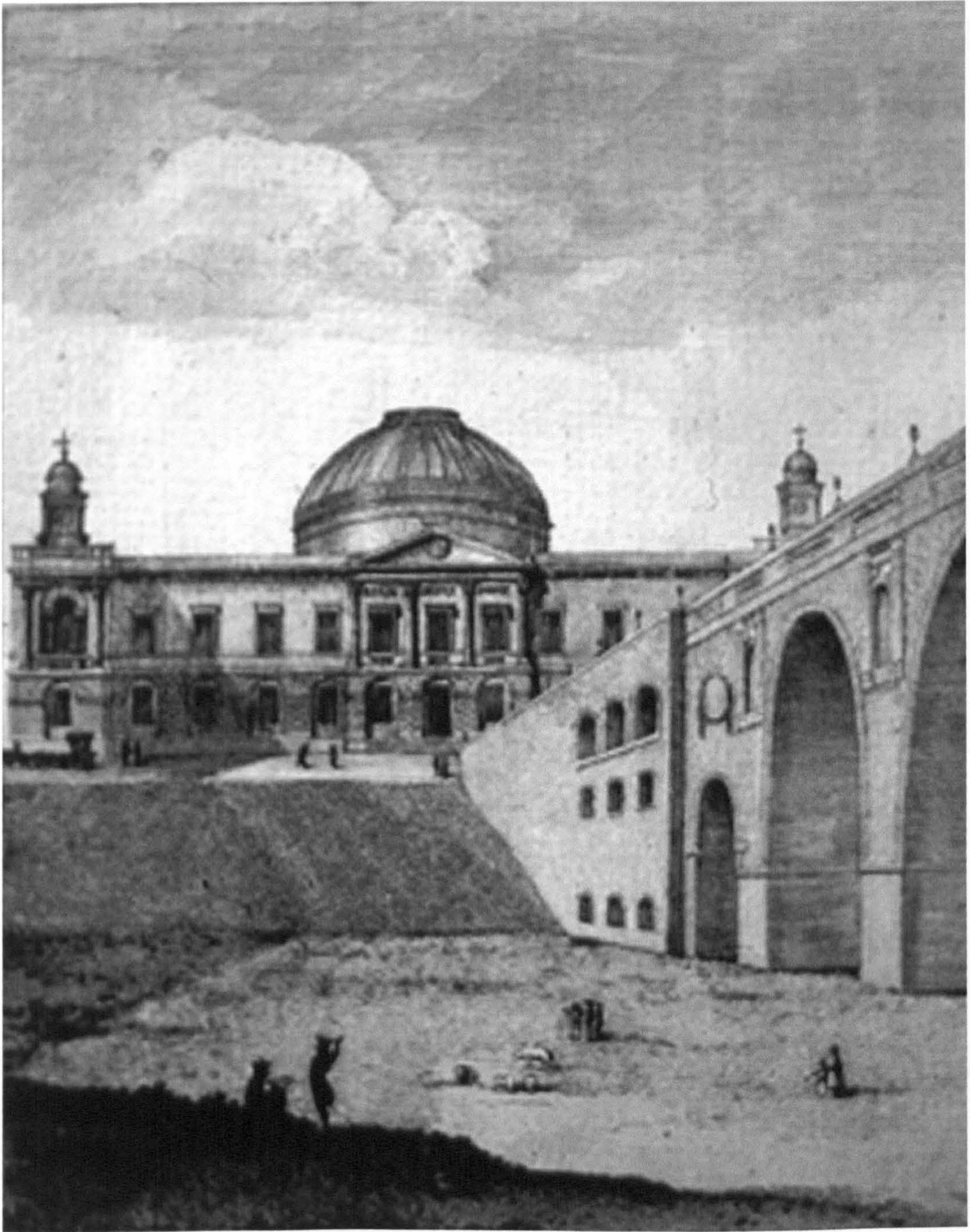
Plate 56: William Mylne, bridge over Nor Loch, 1765
