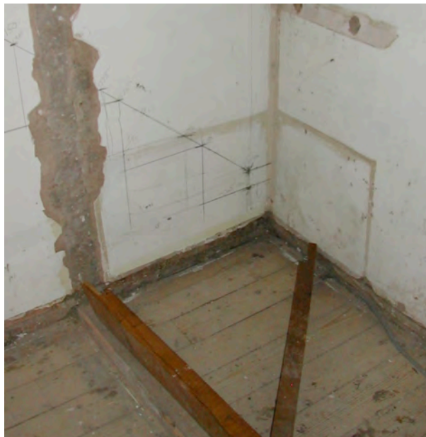
Figure 9.11 Site Markings for the Staircase Winding Steps
