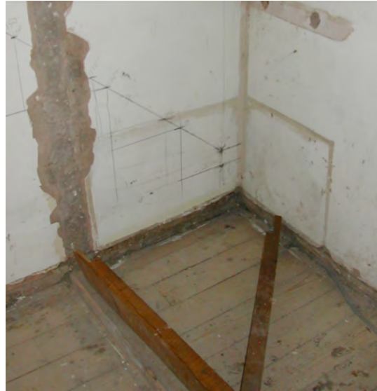
Figure 6.8 Sacred staircase markings on the construction site
