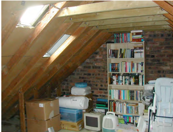
Figure 6.2 Condition of roof space before conversion
