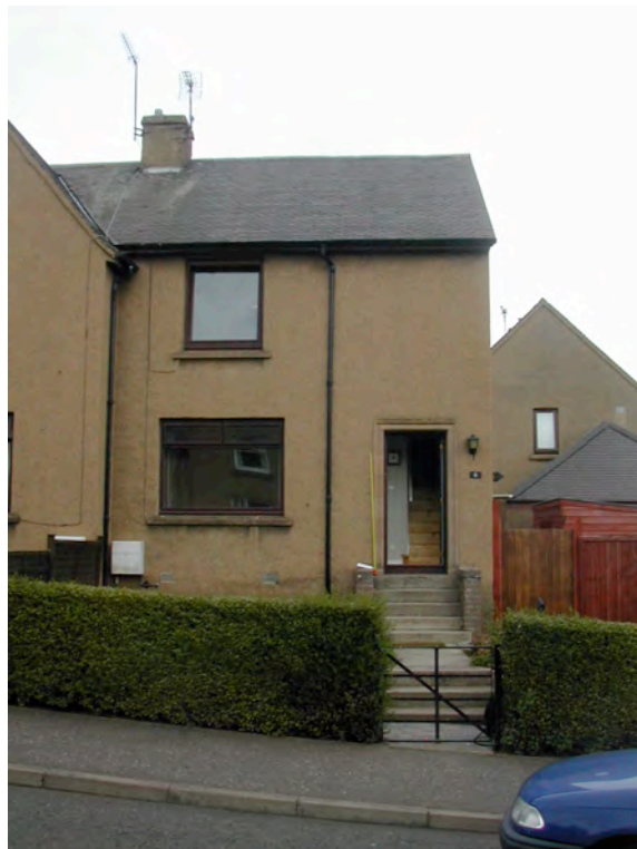
Figure 6.1 House before roof space conversion
