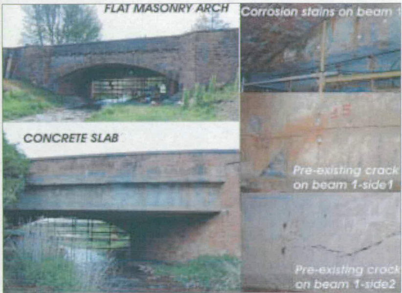
Fig 2. (above) Boghall bridge: masonry and concrete side; pre-existing cracks
