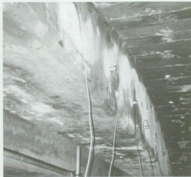
Fig. 21. Sensors fixed on the north side of the west end of the concrete beam.
