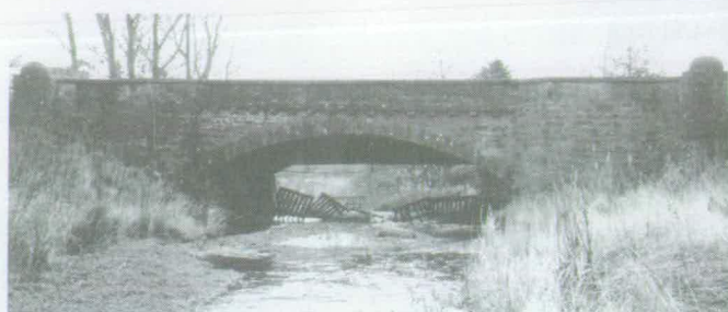
Fig. 1. Boghall Bridge viewed from the north side.
