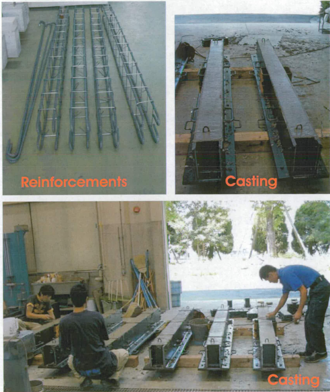
Figure 6.25: Phases of the casting of the beams in Kumamoto Laboratory.
